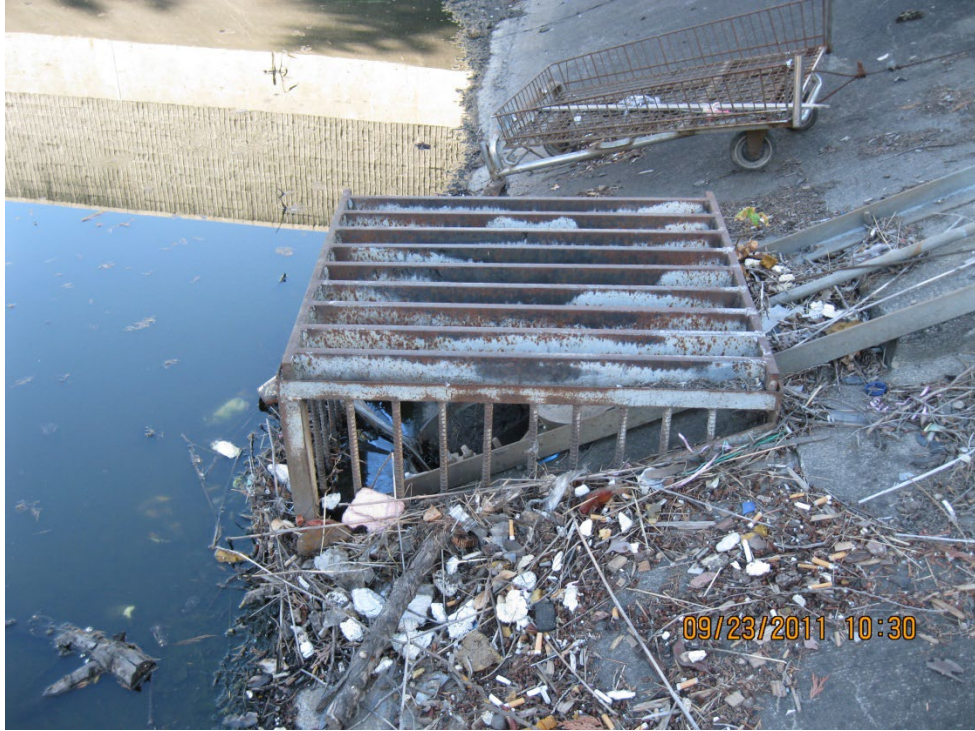
Photo 4: Detention pond outlet with gate.
