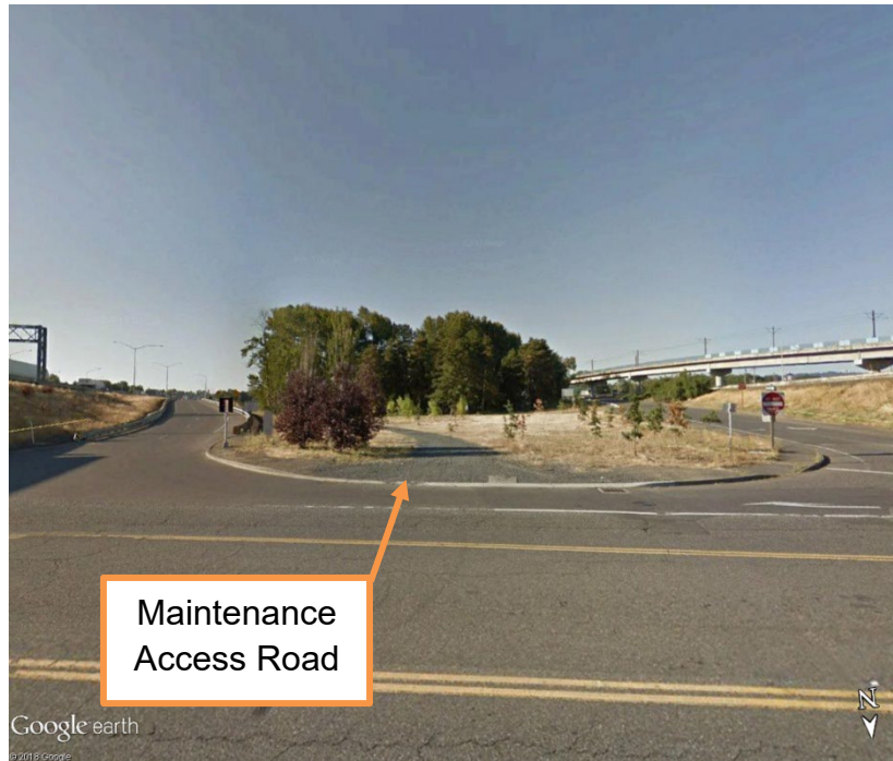
Figure 3: Maintenance Access Road entrance, facing South from N. Victory Blvd.
