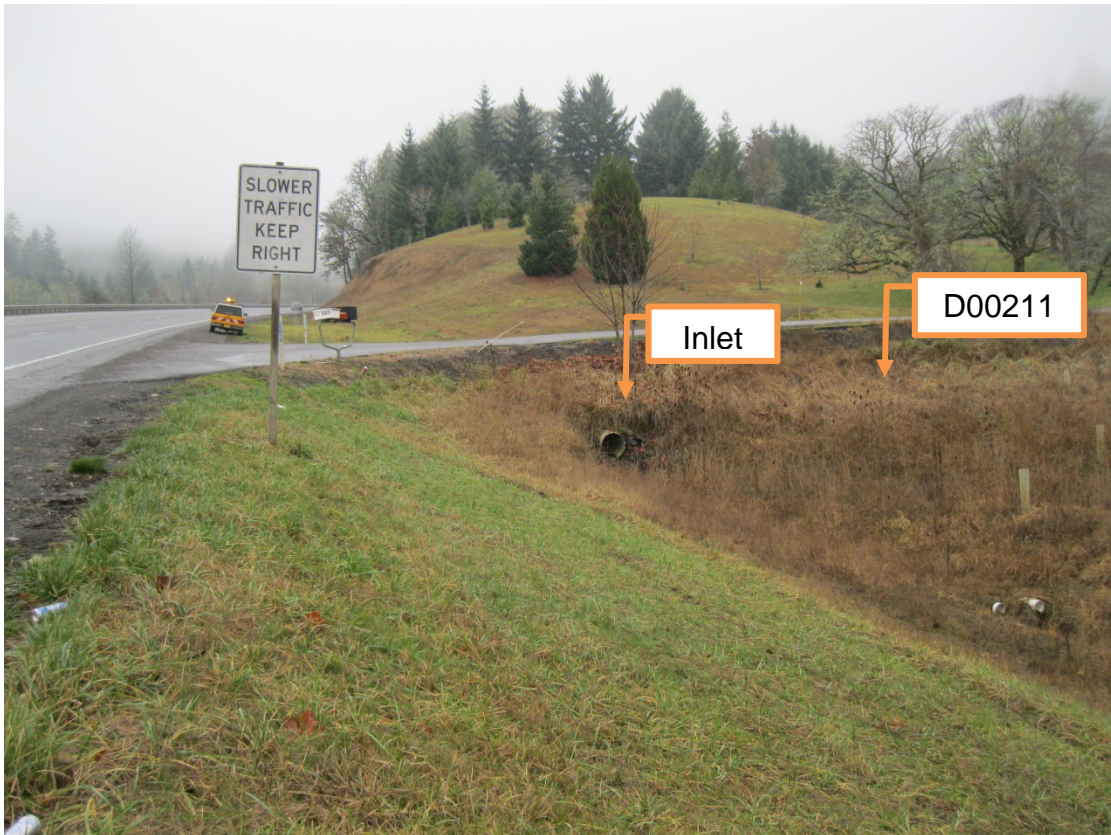
Figure 3: Facility access via roadside shoulder, looking West
