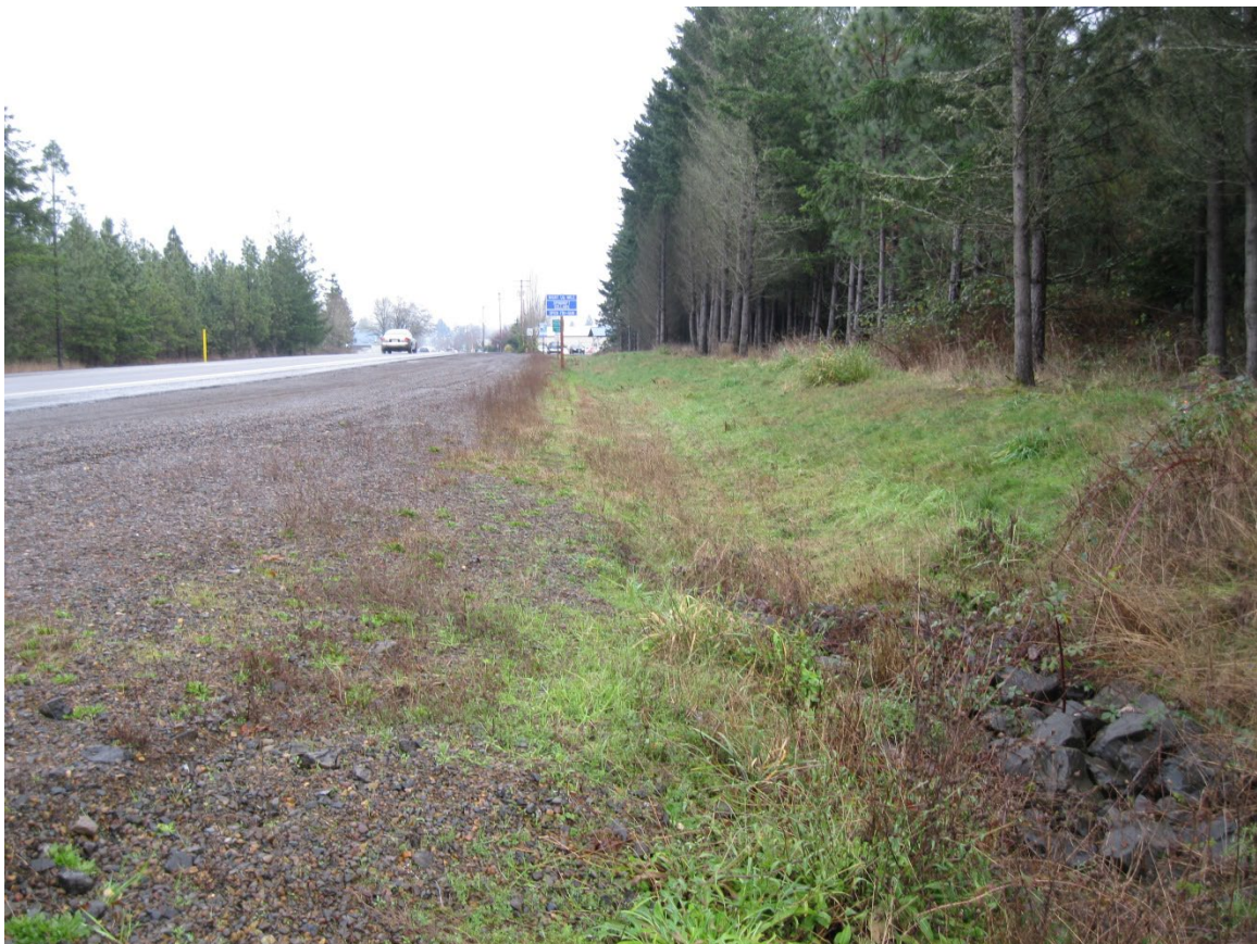
Figure 1: DFI No. D00209, looking East
