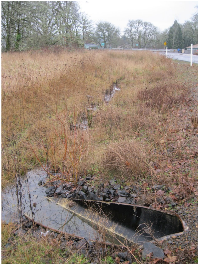
Figure 1: DFI No. D00208, looking Southeast
