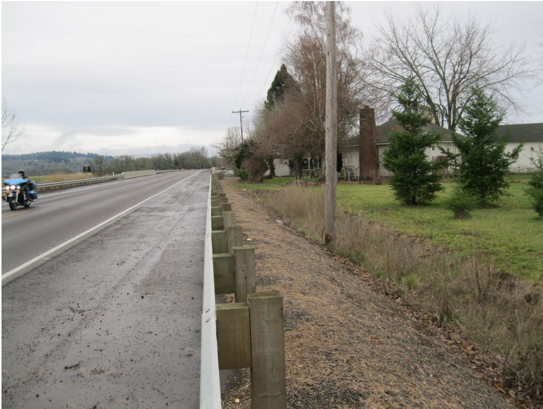
Figure 3: Facility access via roadside shoulder, looking Northwest
