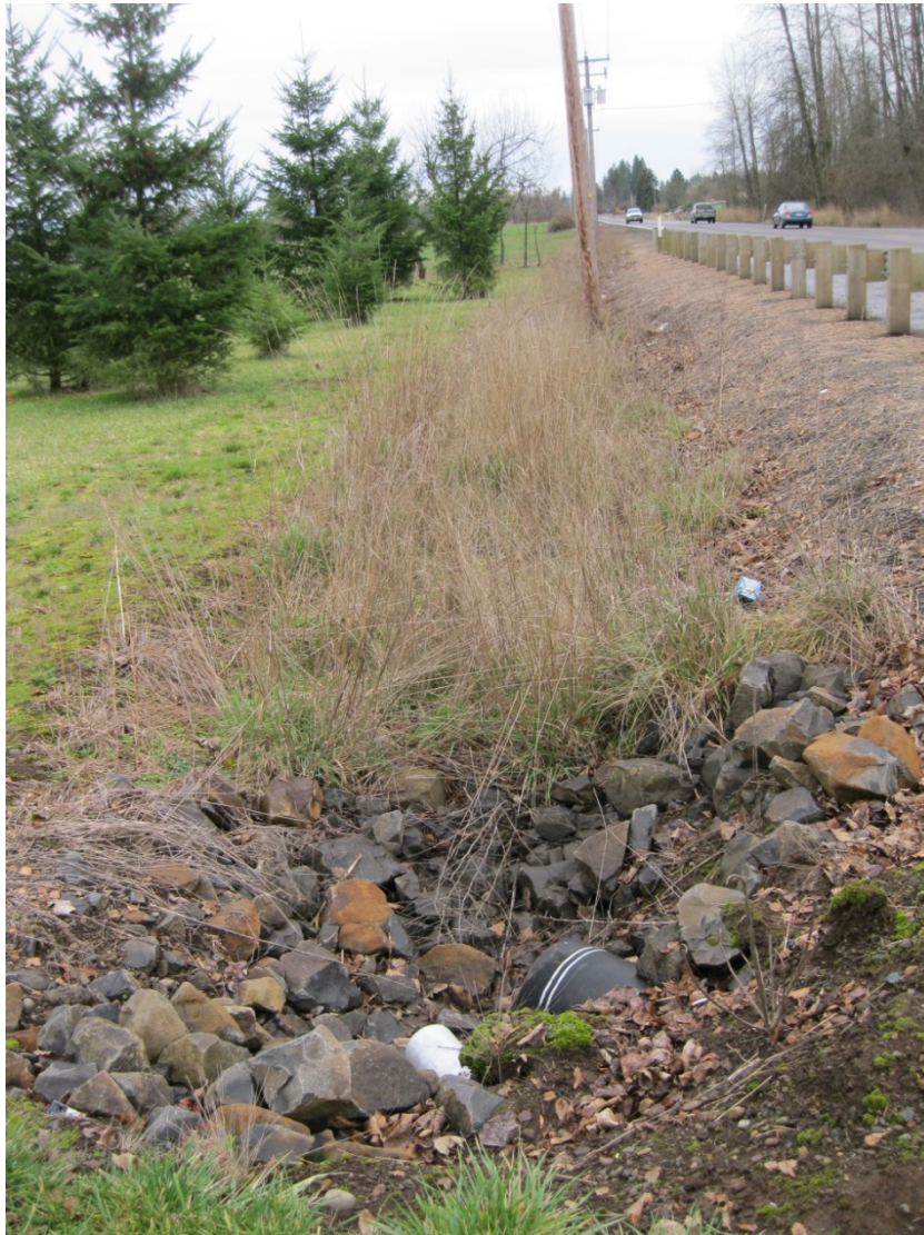
Figure 1: DFI No. D00207, looking Southeast
