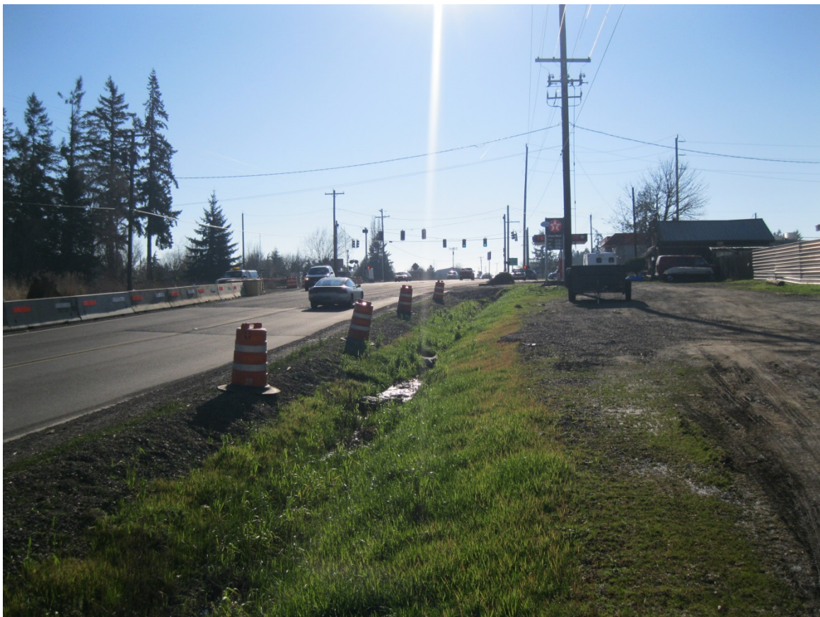
Figure 1: DFI No. D00203, looking South
