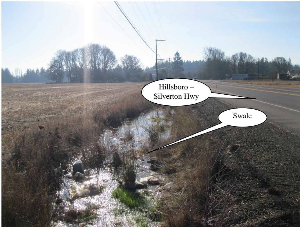
Photo 1: This photo depicts swale and its relative position to Hillsboro-Silverton Highway.
