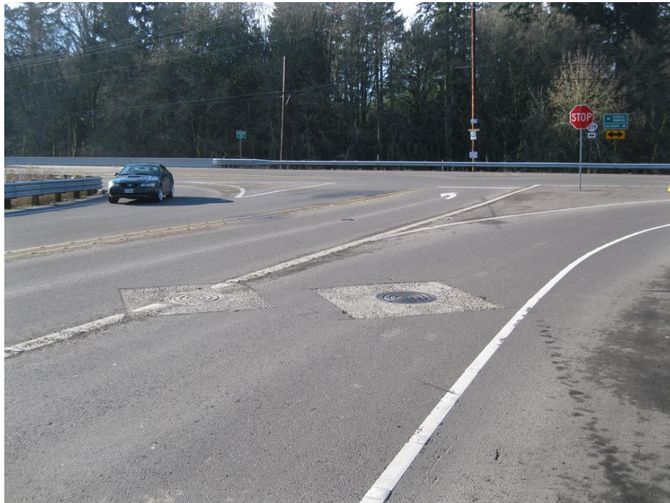
Photo 1: Looking southwest at flow control manhole structure; Point A, Ops Plan.
