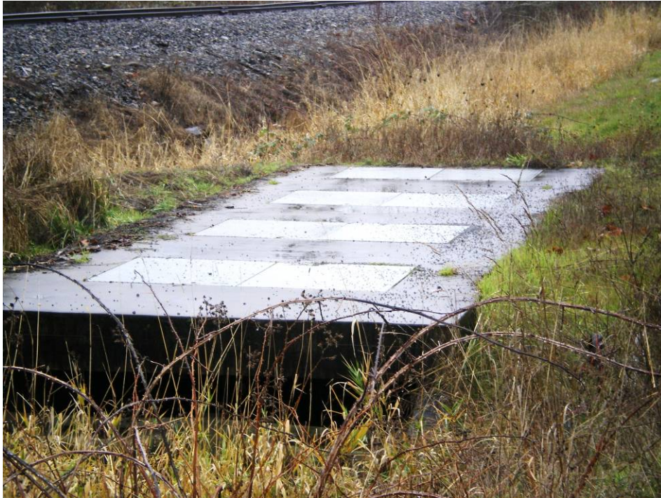
Photo 1: Compost Stormwater Filter looking southeast. US Route 30 is located to the right. The inlet and outlet for the treatment system is shown in the foreground.
