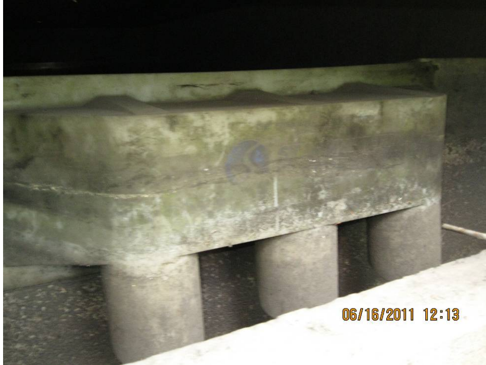
Photo 4: View of the riser pipes and inlet hood as they would convey water to the filter bed.
