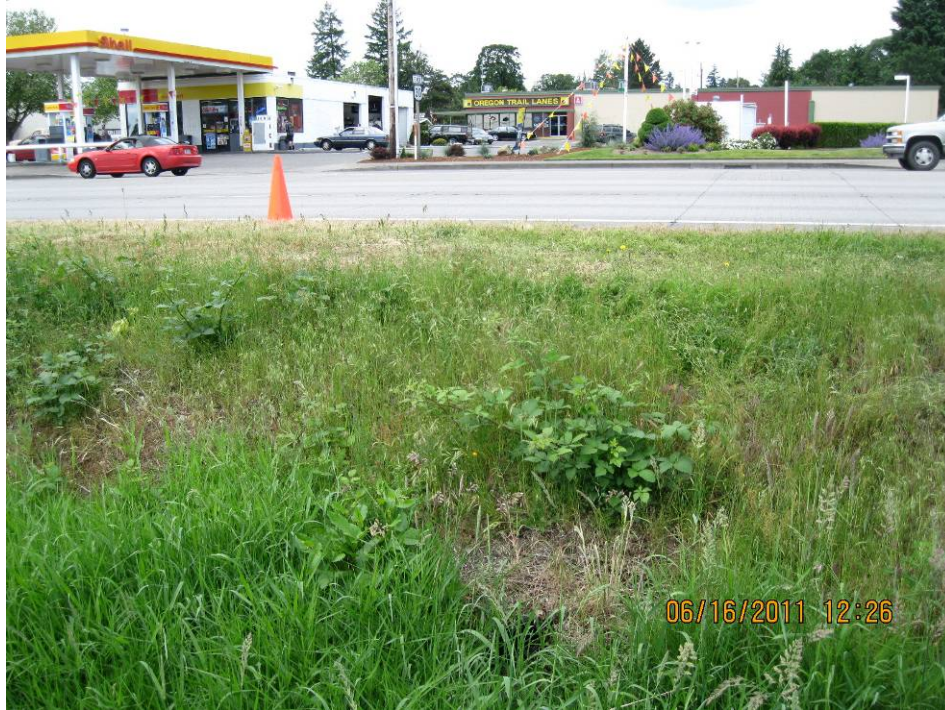
Photo 1: Looking west toward the culvert inlet at Point A –the beginning of the swale.
