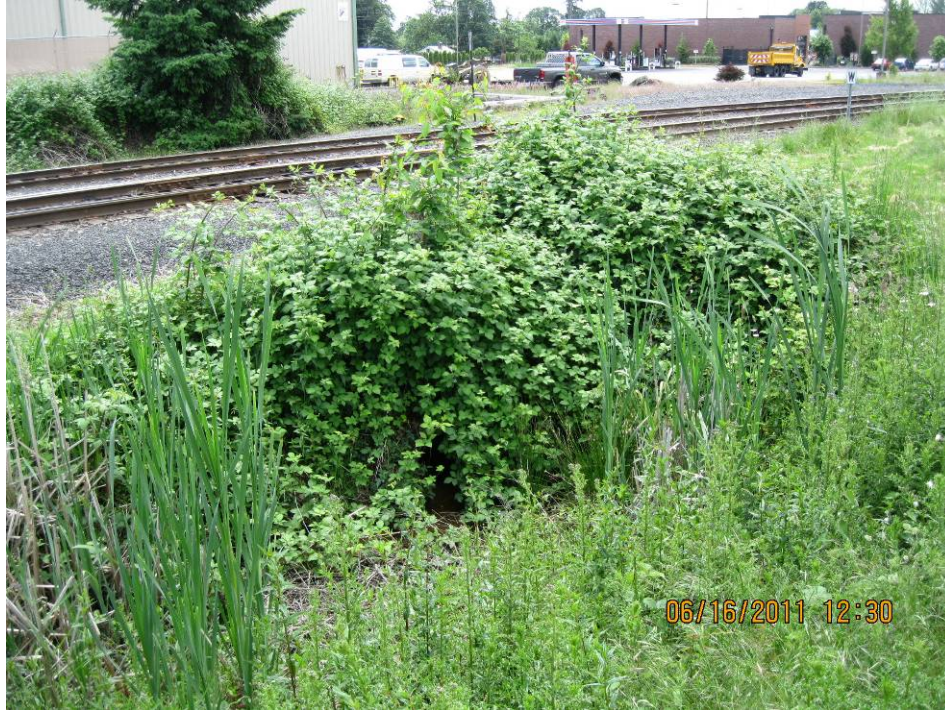
Photo 3: Looking south toward the end of the swale and the facility outlet at Point C.
