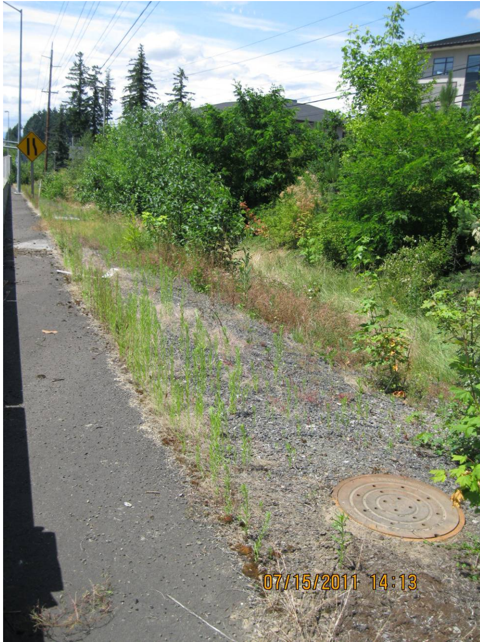
Photo 1: Looking NW at Water Quality Manhole and adjoining swale (D00177).
