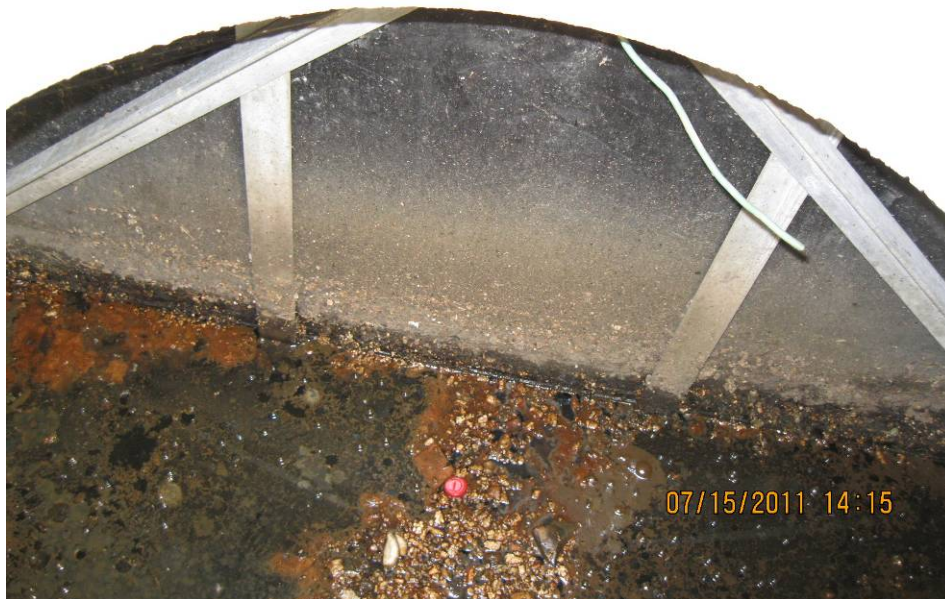
Photo 3: Internal view of Water Quality Manhole.
