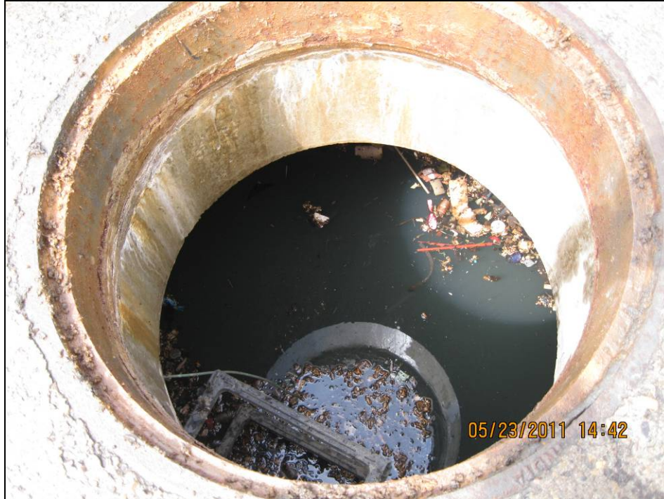
Photo 2: Internal view of Water Quality Manhole.
