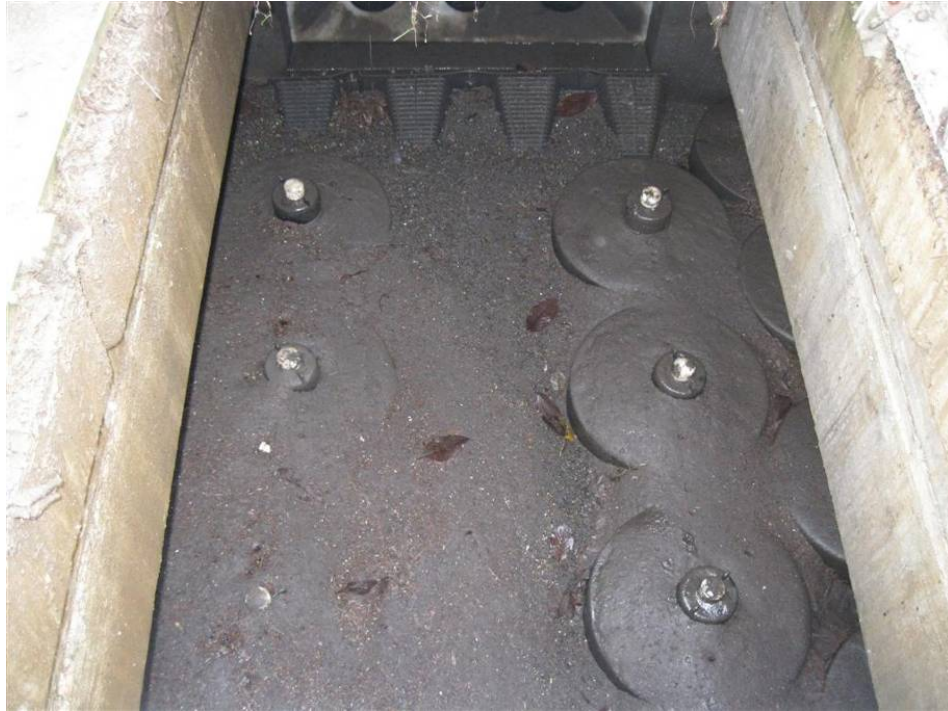
Photo 1: Looking inward at the inlet energy dissipater – facility inlet; Vault 1.
