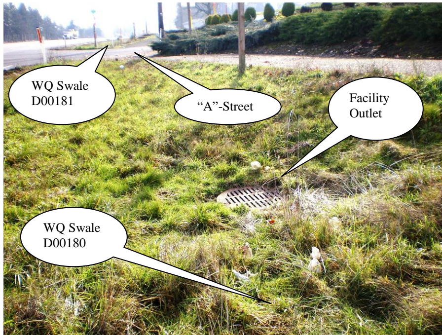
Photo 3: Looking south toward "A"-Street and the facility outlet.
