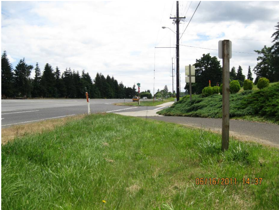
Photo 2: Looking south toward Hwy. 92 and D00181 Swale beyond "A" Street.
