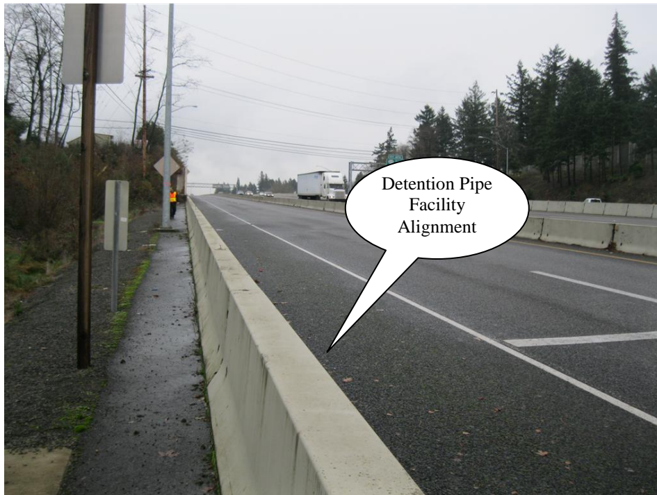
Photo 2: Looking east along detention pipe facility alignment. Water Quality Facility DFI D00177 is located to the left.
