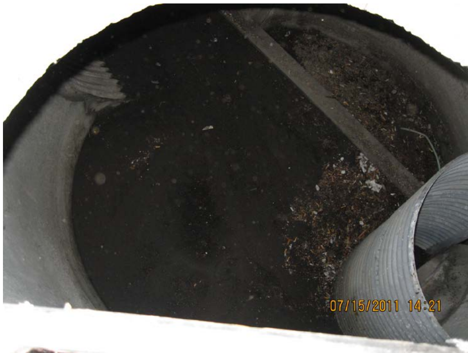
Photo 4: Looking inside of the flow control manhole at the terminus of the detention pipe facility; Point D on Operational Plan; Appendix A.
