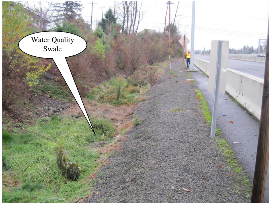
Photo 5: Water quality swale looking east. US 26 (Hwy 047) is located to the right.
