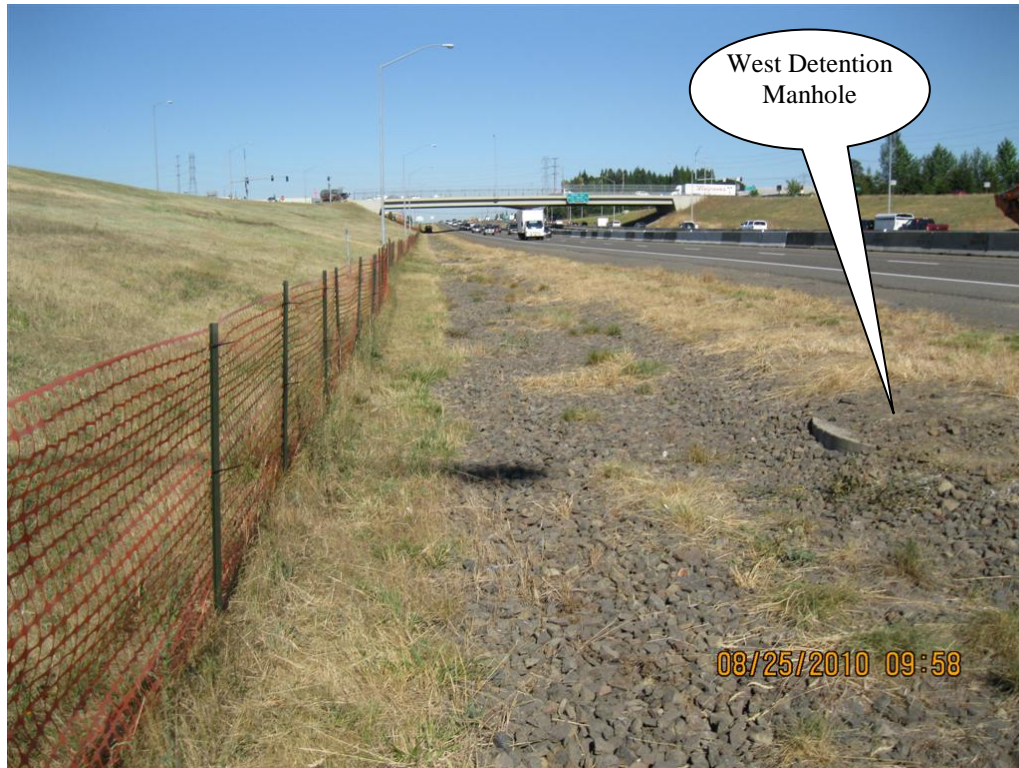
Photo 1: West manhole of the detention facility. Photograph is looking west with US 26 (Hwy 047) to the left.
