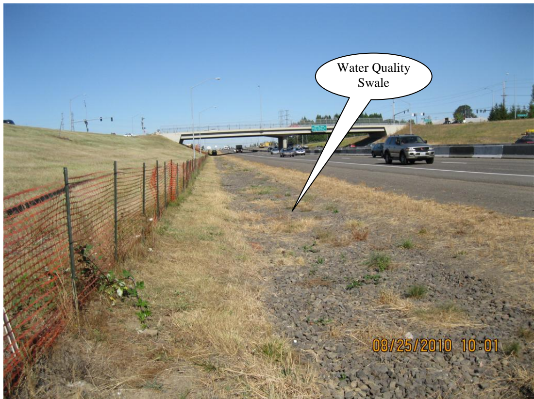
Photo 4: Water quality swale looking west. US 26 (Hwy 047) is located to the right.
