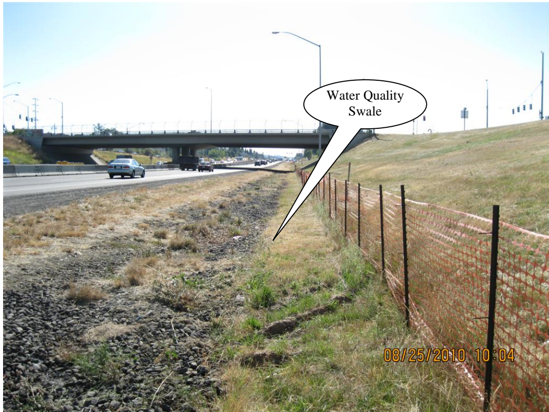
Photo 1: Water quality swale looking east. US 26 (Hwy 047) is located to the left.
