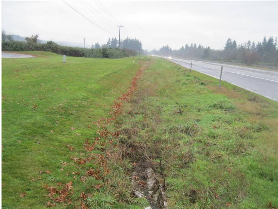
Photo 1: Looking north at water quality swale. Hwy 92 is located to the right.
