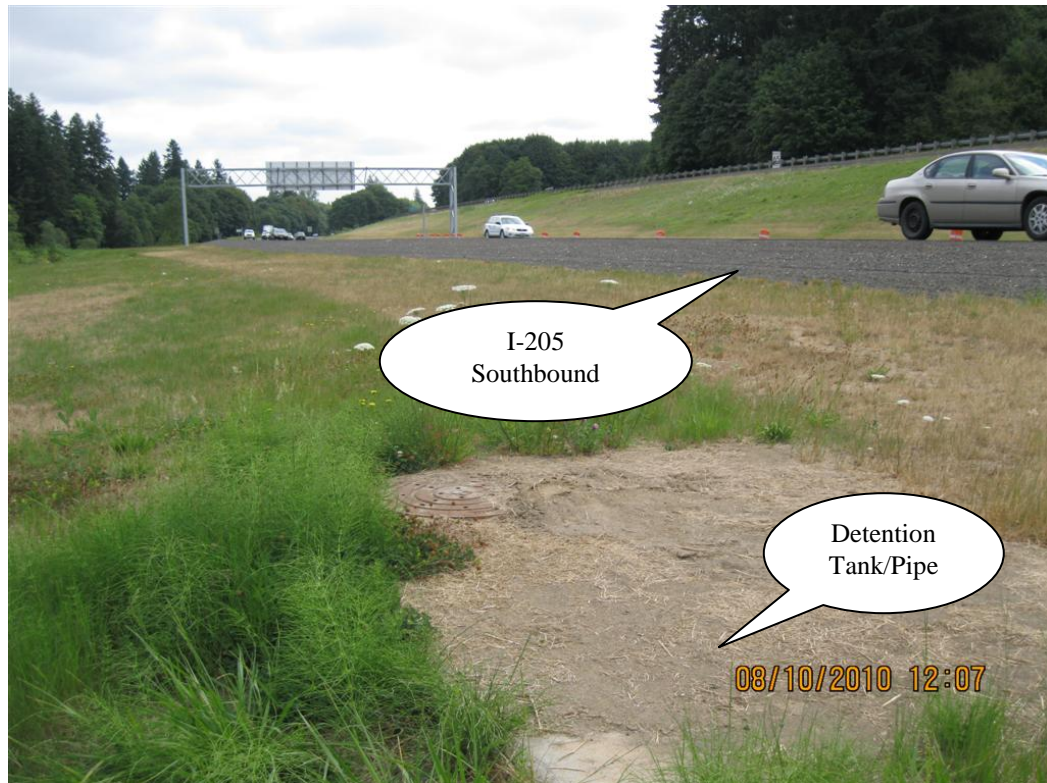
Photo 1: Detention Tank/Pipe along I-205 (Hwy 064) Southbound.
