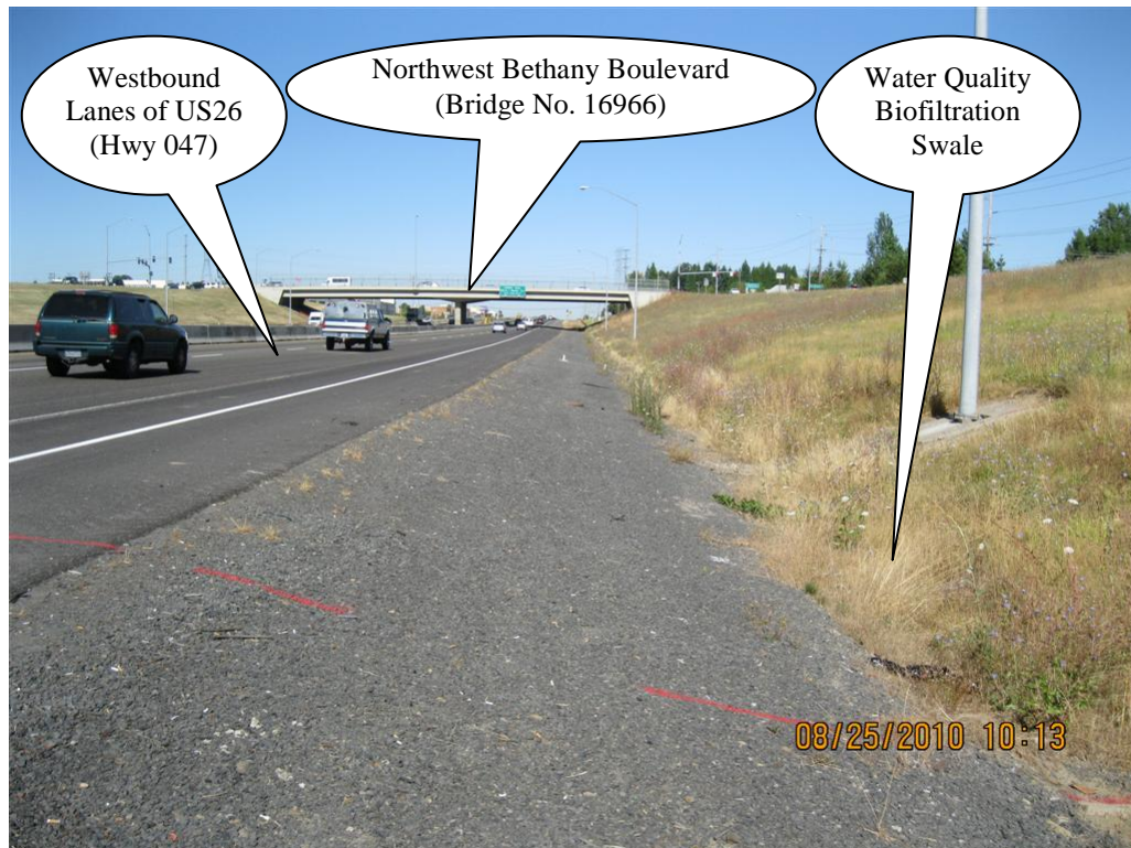
Photo 1: Water quality biofiltration swale. Westbound lanes of US26 (Hwy 047) are on the left. Photo taken facing west.
