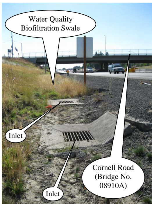
Photo 5: Two of three inlets ( Points B, C ). Photo taken facing east.
