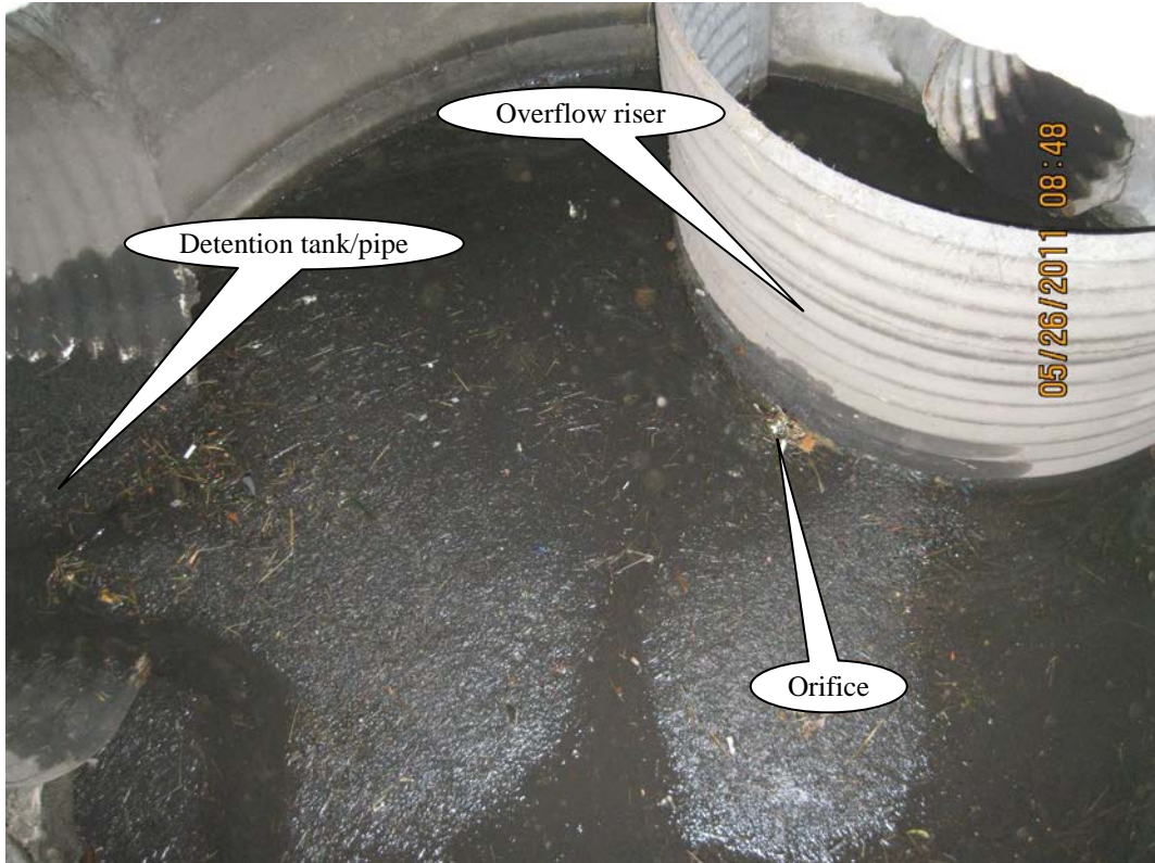
Photo 2: Flow control manhole
