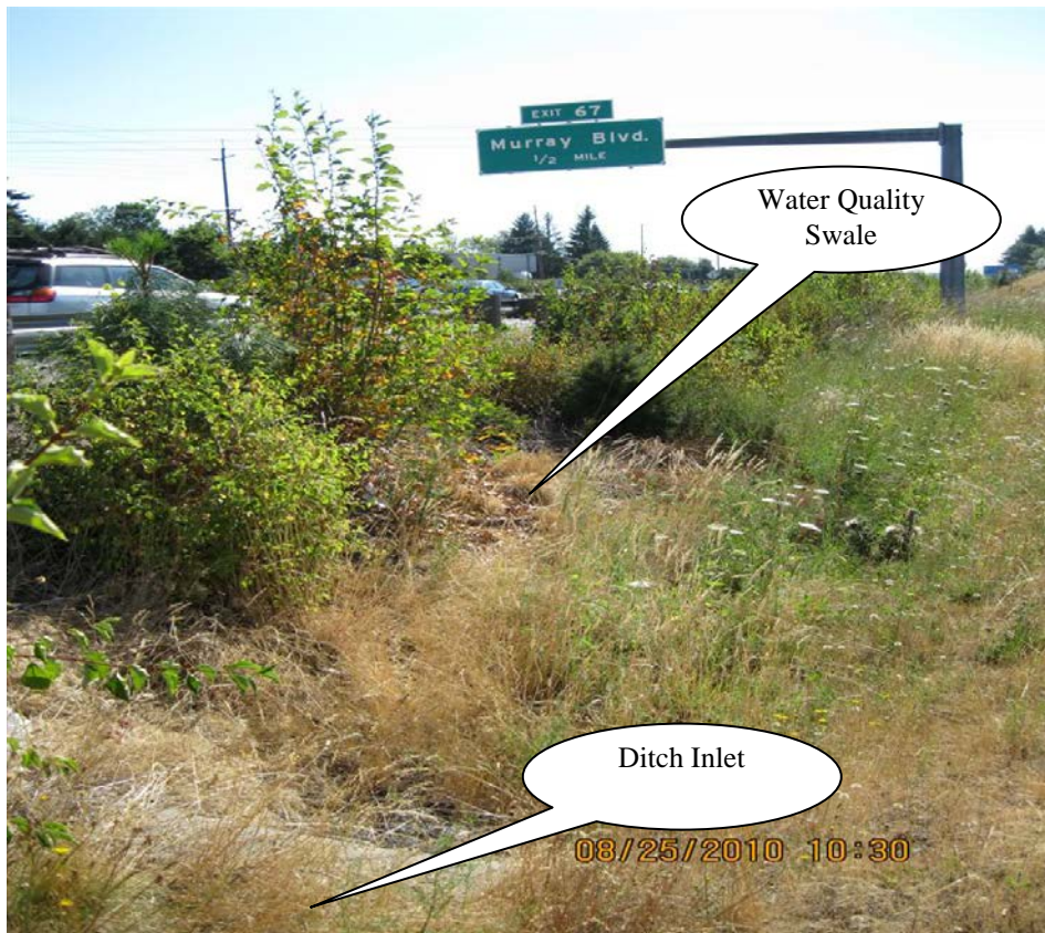
Photo 2: Water quality swale looking east.
