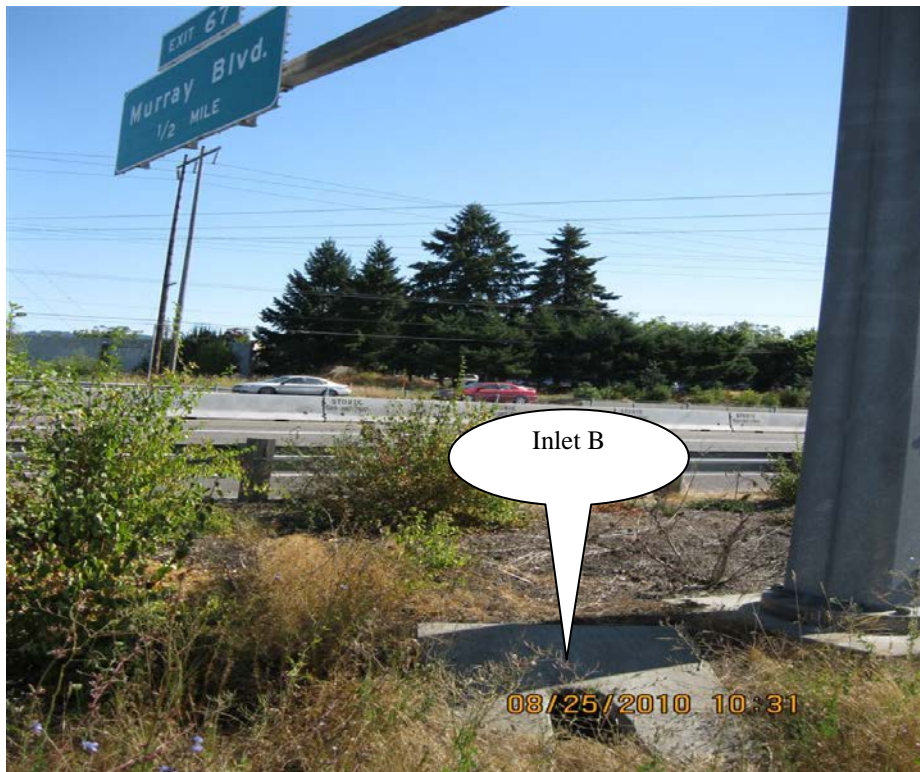
Photo 4: Inlet B to water quality swale.
