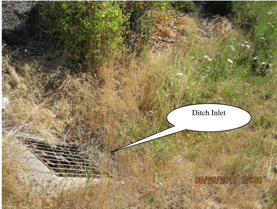
Photo 3: Ditch inlet serving as swale outlet (Point E).
