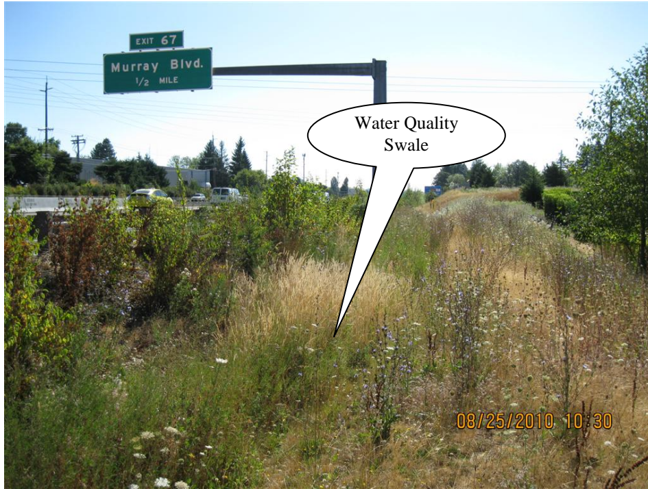
Photo 1: Water quality swale looking east.
