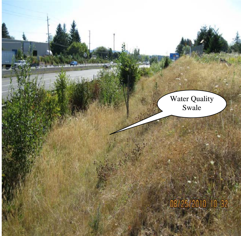
Photo 2: Water quality swale looking towards the east along US26 (Hwy 047).
