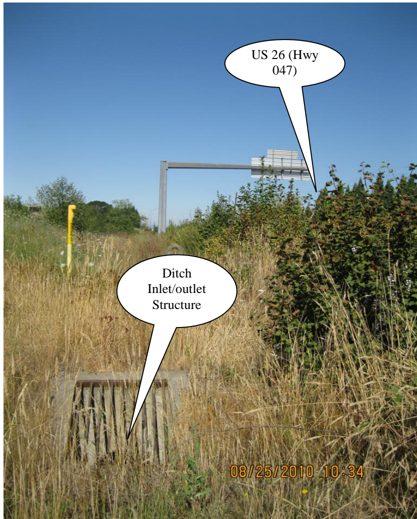
Photo 1: Ditch inlet structure serves as the facility outlet.
