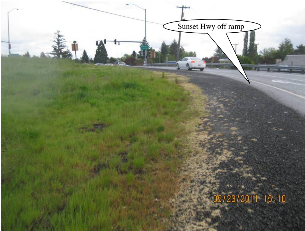
Photo 2: Swale looking south
