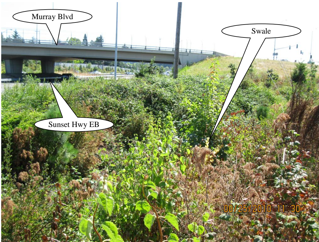
Photo 4: Water quality swale looking towards the east.
