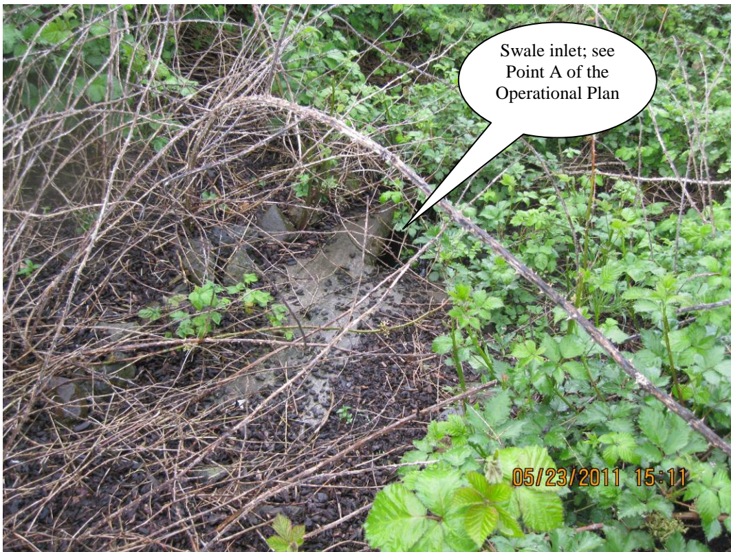
Photo 5: Swale inlet looking south
