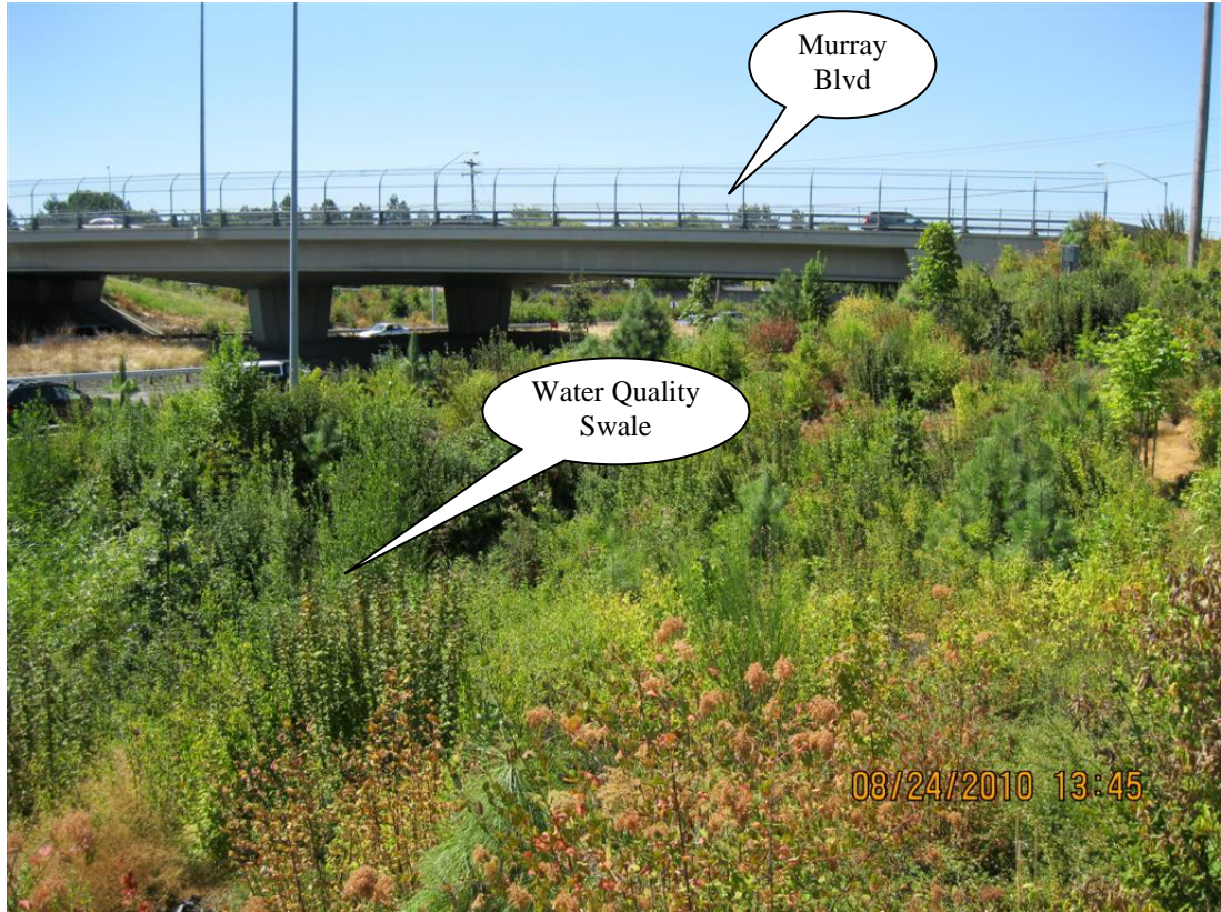
Photo 1: Water quality swale looking towards the west at the Murray Blvd overpass on US 26.
