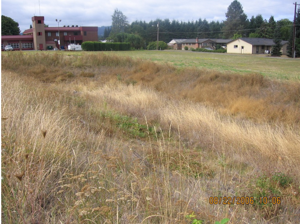
Photo 4: Water quality biofiltration swale. Photo taken facing south.
