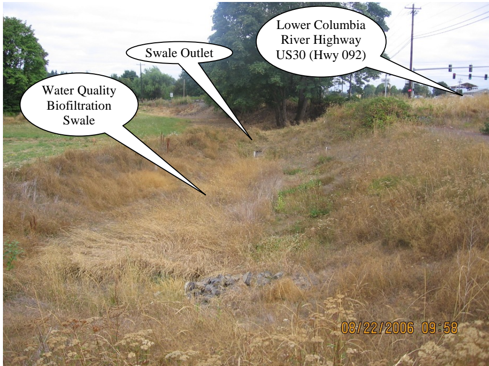
Photo 2: Water quality biofiltration swale. Photo taken facing north toward the swale outlet.
