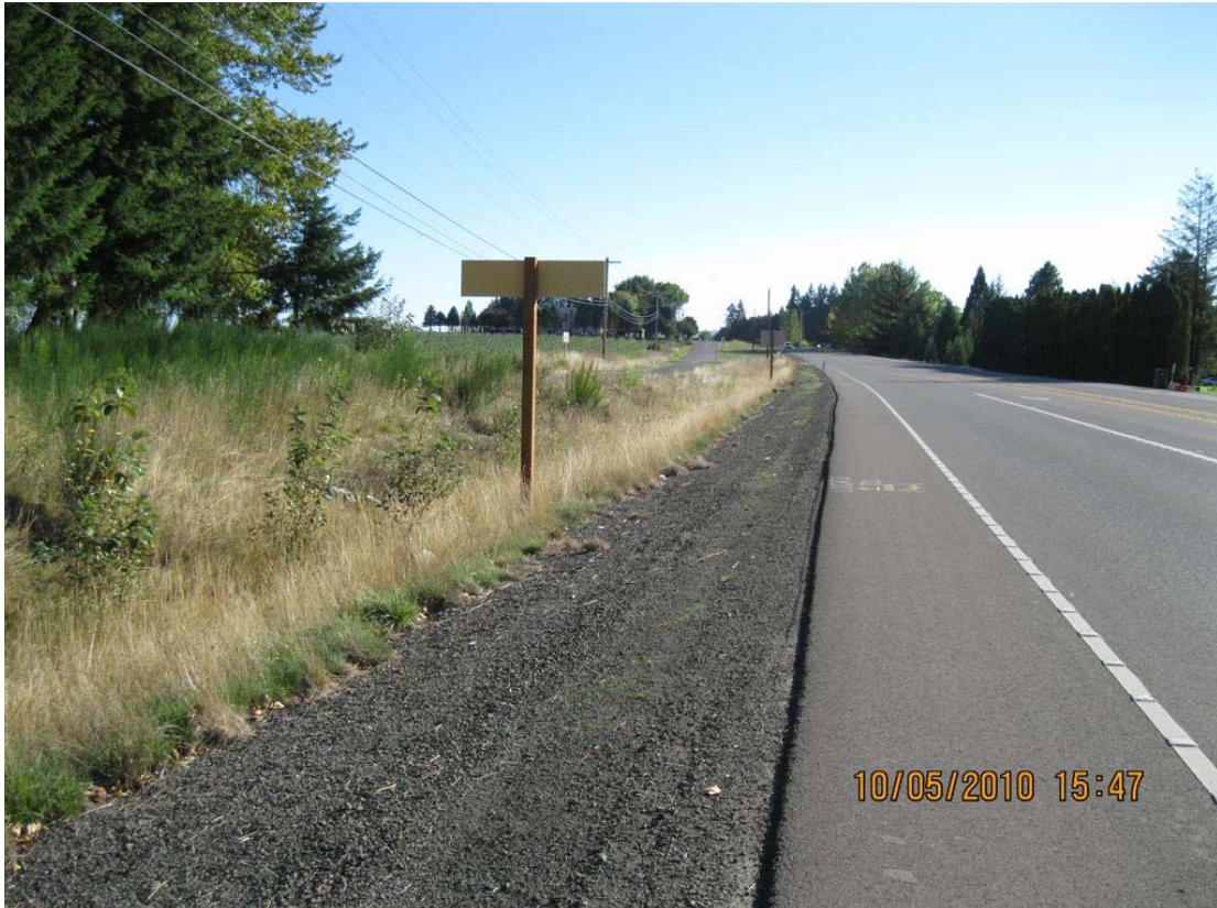
Figure 3: Swale facility with shoulder access, looking South
