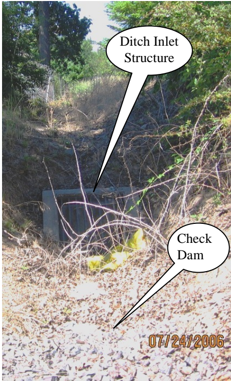
Photo 3: Ditch inlet structure near the north end of the swale.
