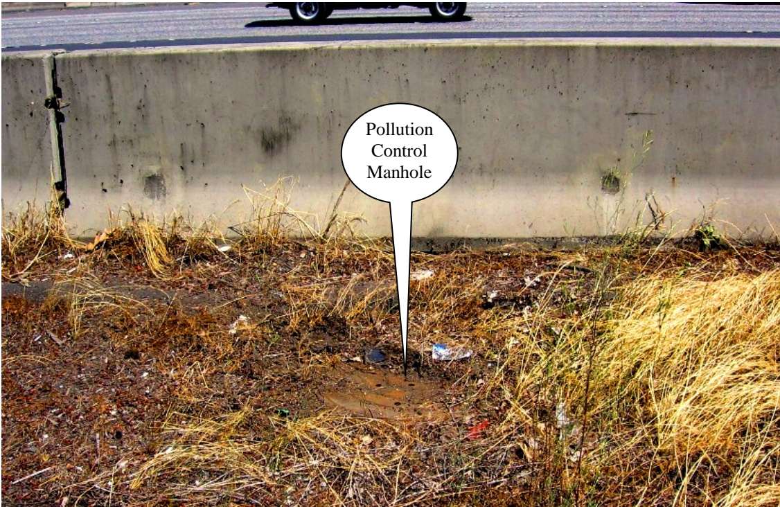
Photo 2: Pollution control manhole near the south end of the swale.
