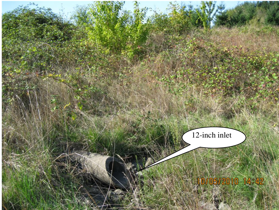
Photo 3: Looking north at the 12-inch diameter facility inlet to the WQ biofiltration swale. I-5 is located to the right.
