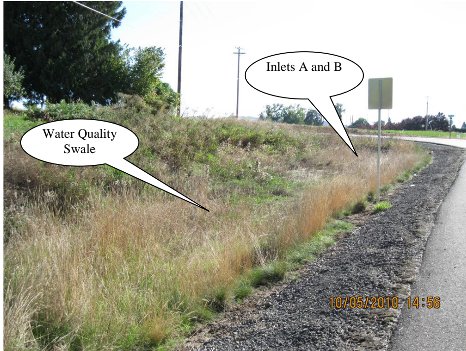
Photo 1: Looking south towards the water quality biofiltration swale and the facility inlets A and B; see the Operational Plan, Appendix A.
