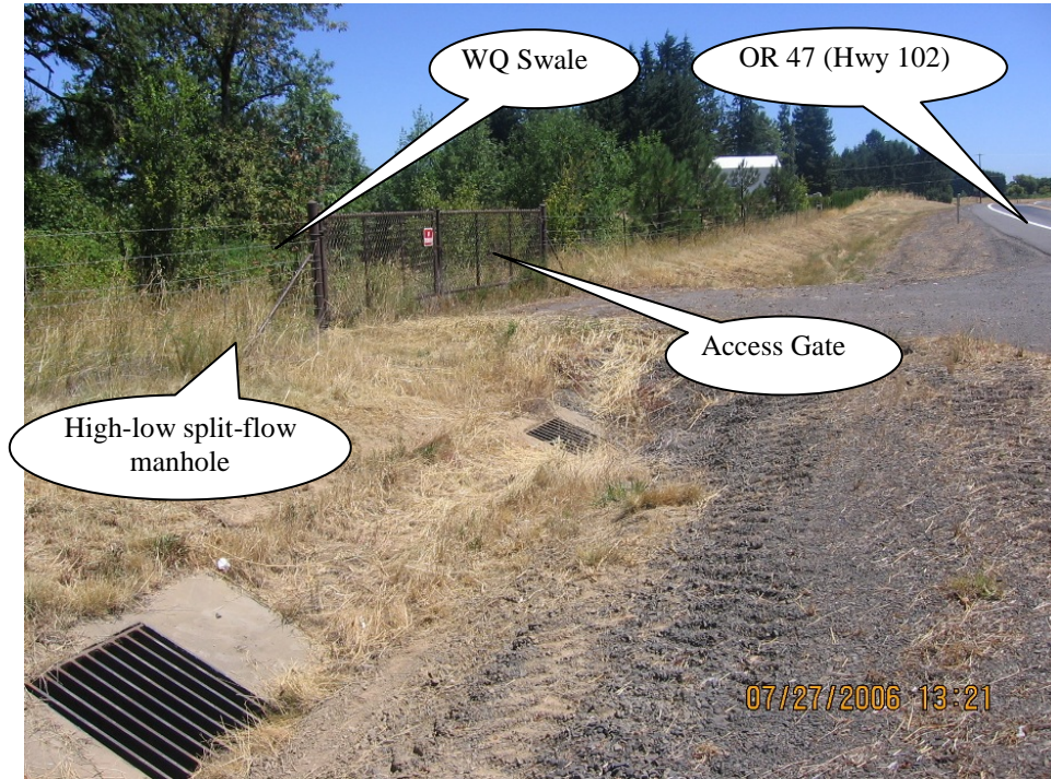
Photo 1: Looking east at inlets along OR 47 (Hwy 102). WQ Swale and WQ Manhole are located within the Access Control Area on the other side of the fencing.
