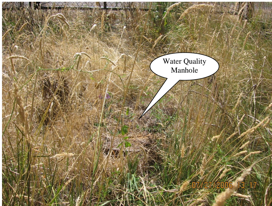
Photo 2: Water Quality Manhole located within Access Control Area.
