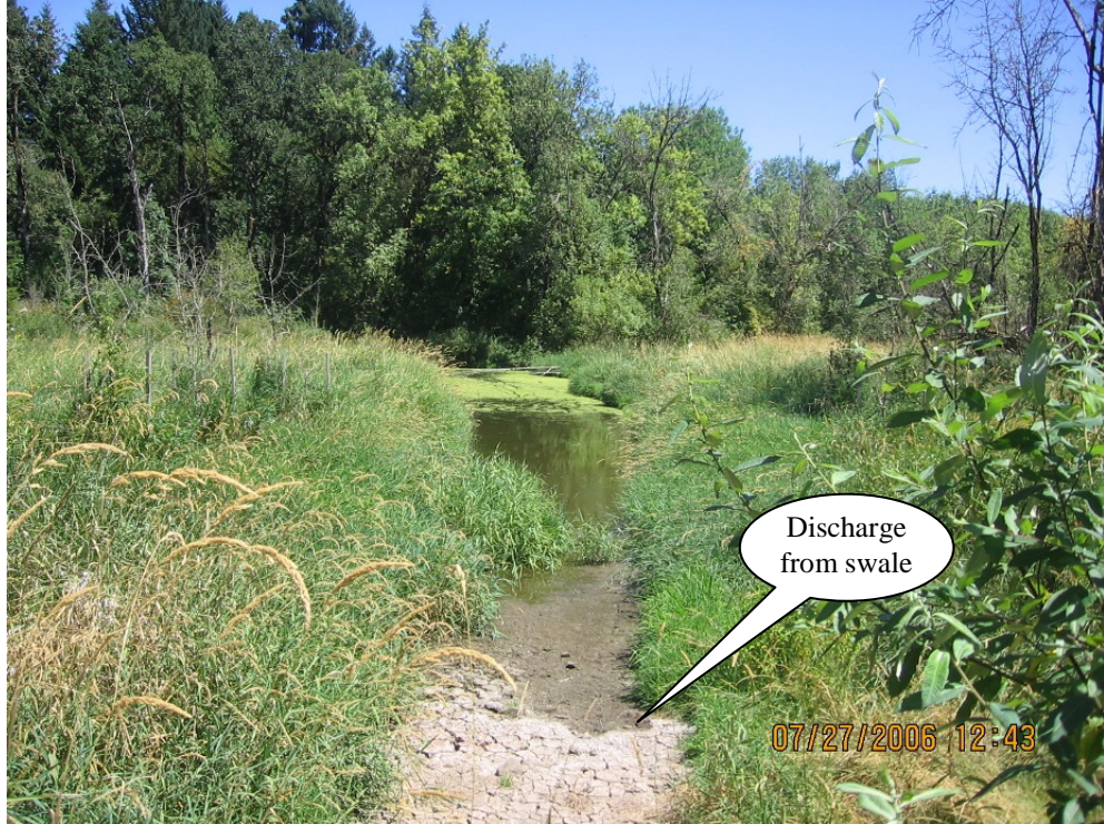
Photo 3: Outlet to WQ Swale discharge into Council Creek. Photograph is looking northeast.
