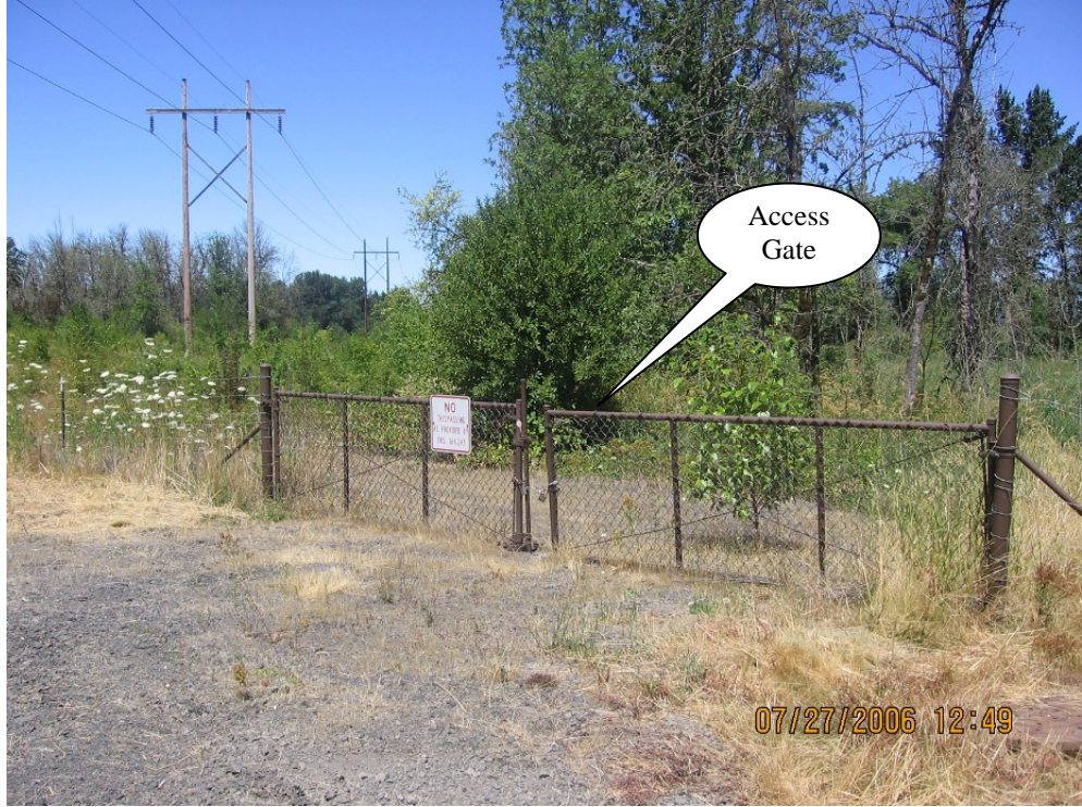
Photo 5: Access gate to WQ biofiltration swale.
