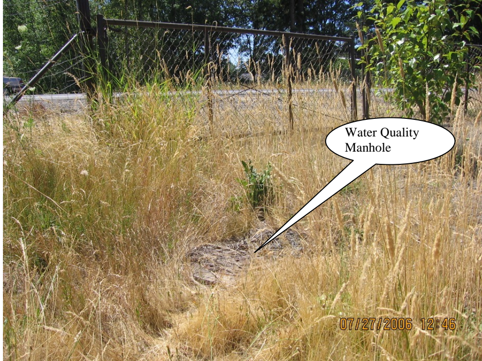
Photo 7: Water Quality manhole located within the Access Control Area.
