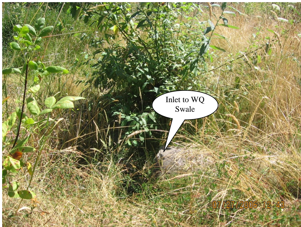
Photo 2: Inlet to WQ swale. Pipe is a 12-inch concrete culvert.
