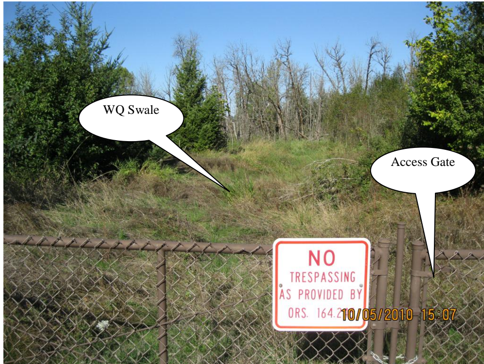
Photo 1: WQ biofiltration swale within Access Control Area. Council Creek is located at base of tree line.
