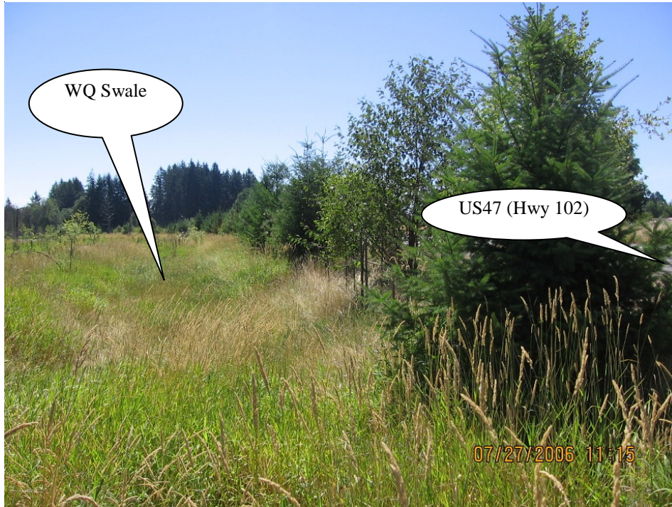
Photo 1: WQ biofiltration swale within Access Control Area. Photograph looking towards southeast.
