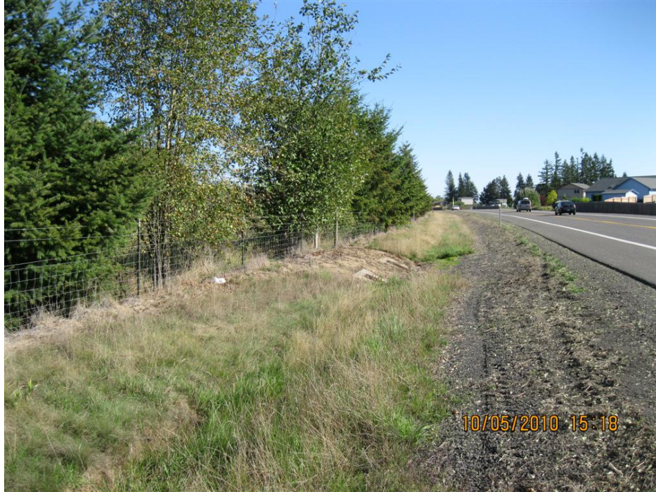
Photo 3: Looking southeast at the roadside drainage ditch with drainage inlets, above.
