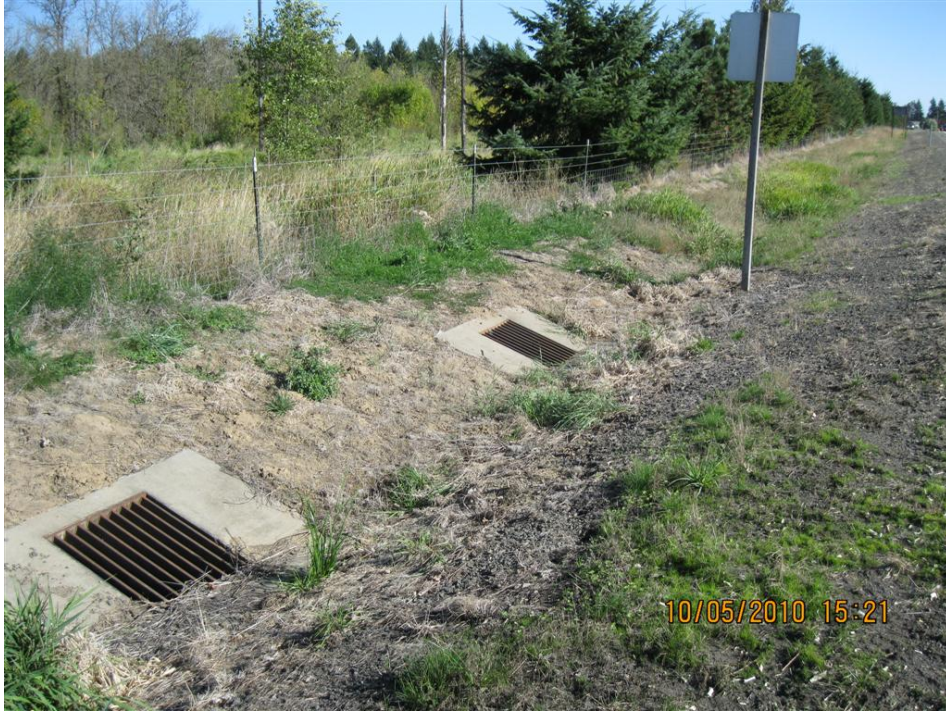
Photo 3: Looking southeast at inlets located along the north side of highway.
