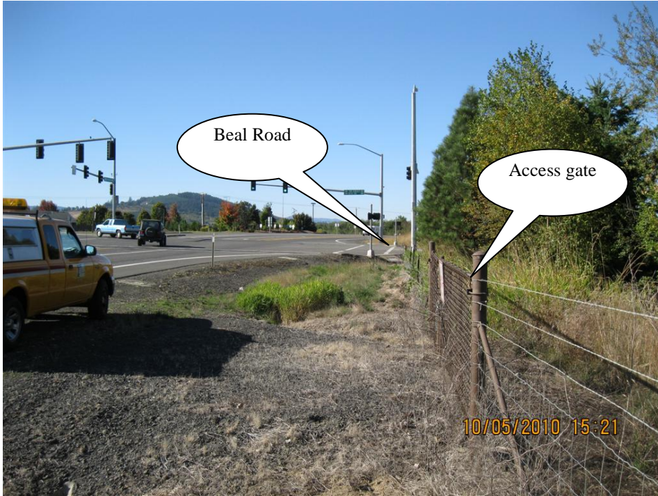
Photo 4: Looking northwest at the access pullout and intersection of US47 (Hwy 102) and Beal Road.
