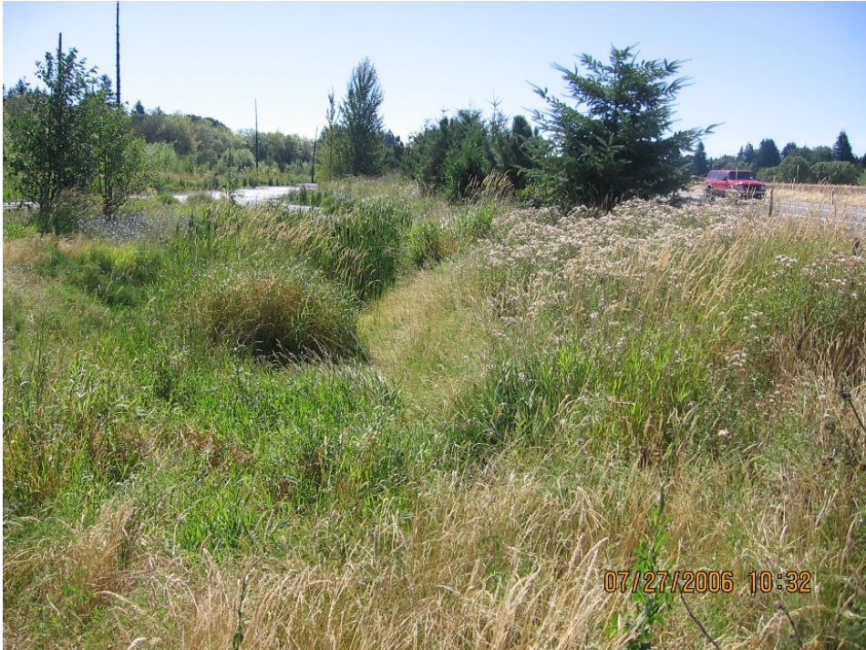
Photo 1: Looking towards the east at the WQ biofiltration swale within the Access Control Area. Council Creek is shown to the left while US47 (Hwy 102) is to the right.
