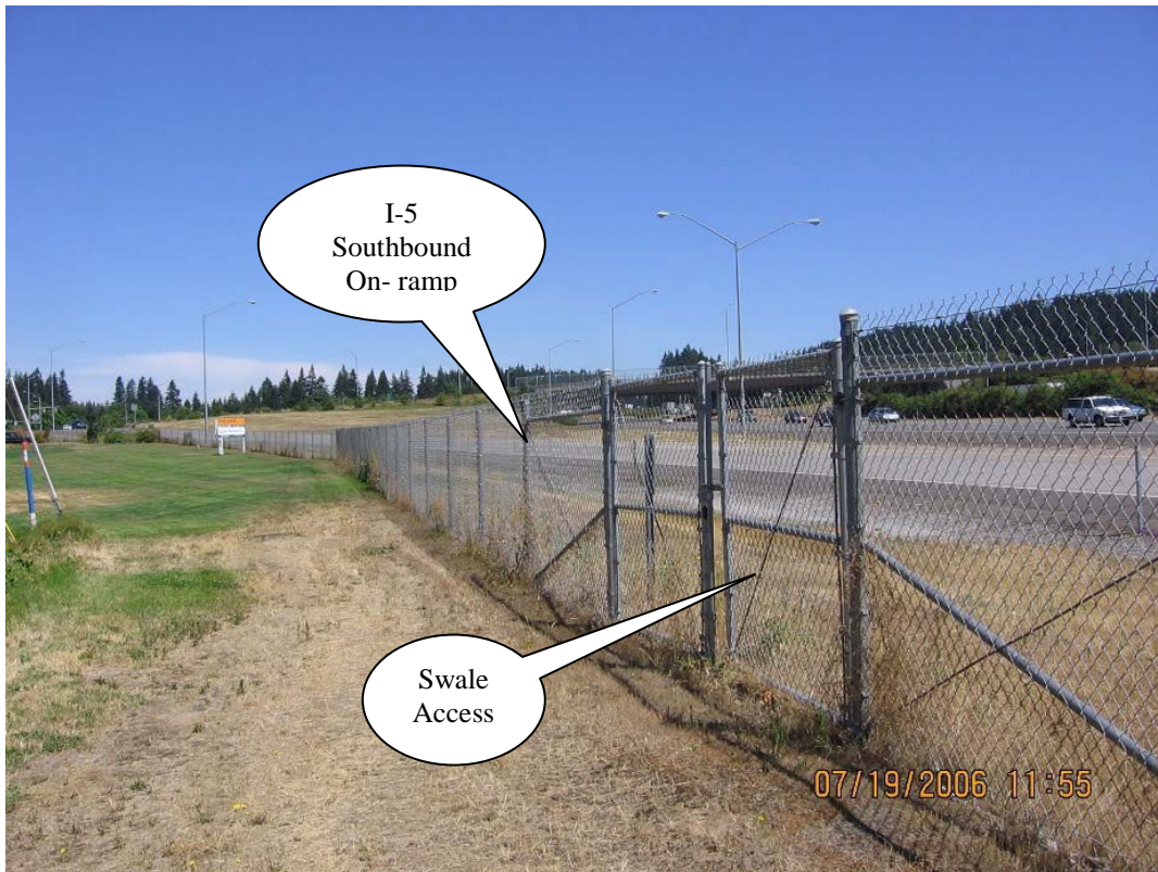
Photo 4: Swale access (looking north)
