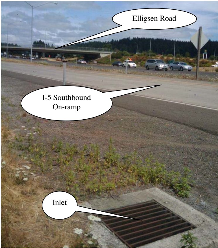
Photo 2: Inlet along the southbound on-ramp
