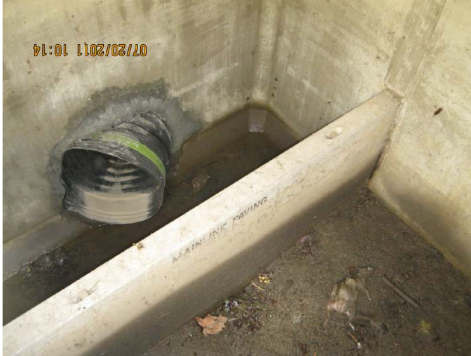
Photo 2: Looking down into outlet vault, Point E, Operational Plan.
