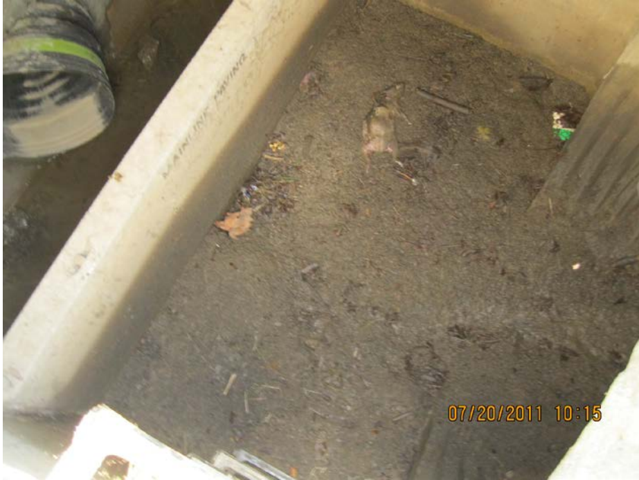
Photo 1: Looking down into outlet vault, Point E, Operational Plan.
