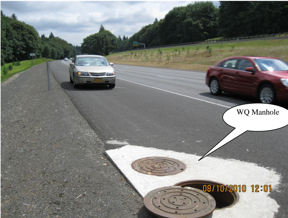
Photo 4: Photo looking east towards the southbound travel lanes. The WQ Manhole is in the foreground.
