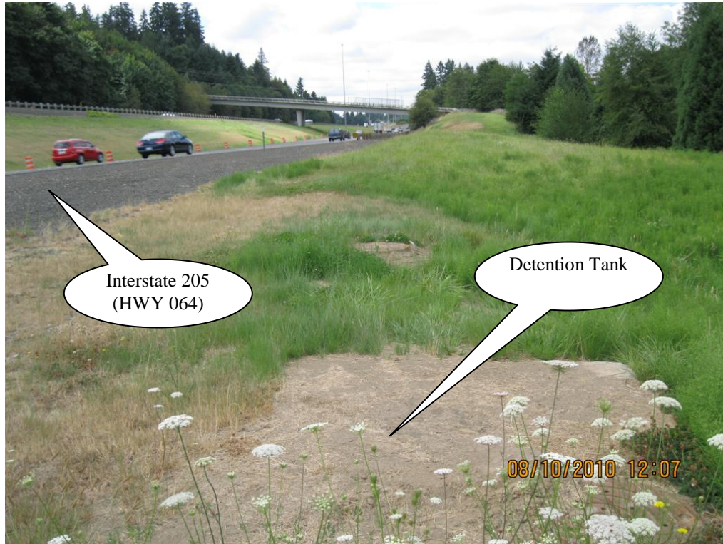
Photo 1: Looking west at the buried detention tank/pipe system.
