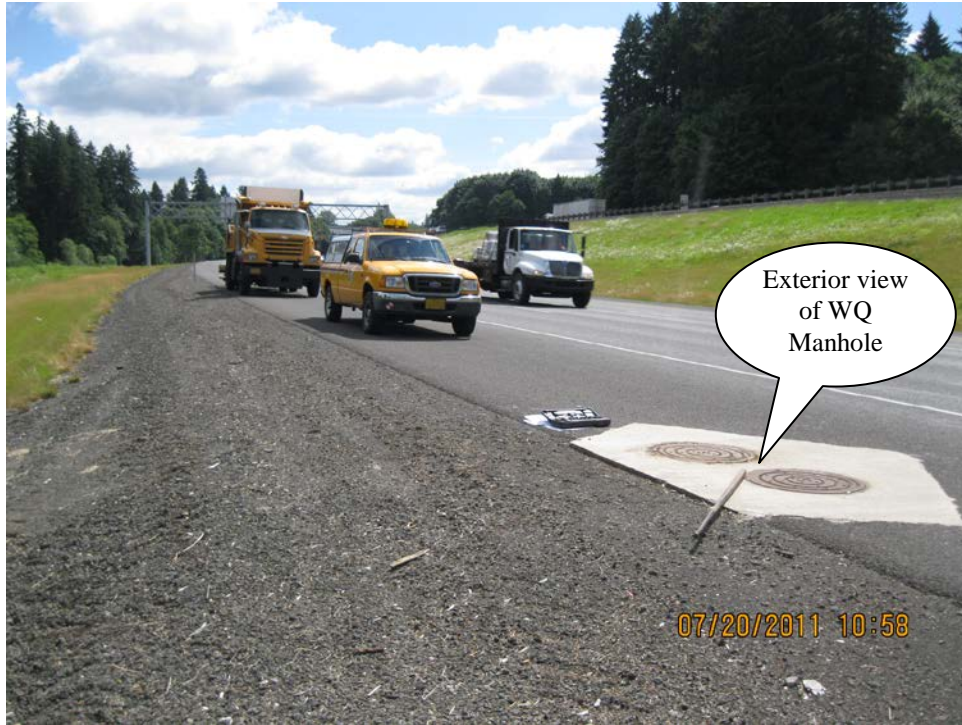
Photo 1: Looking southeast at water quality manhole (CDS Unit) covers and SB I-205.
