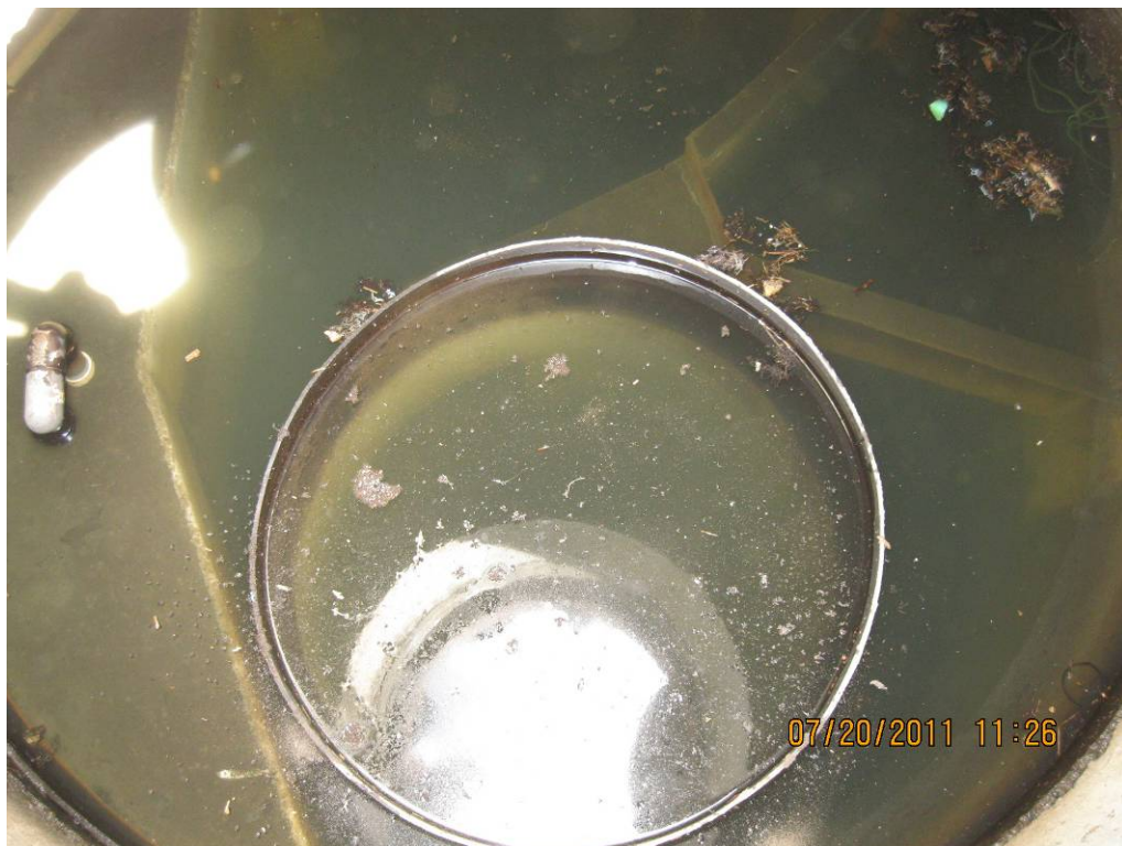
Photo 2: Internal view of water quality manhole.
