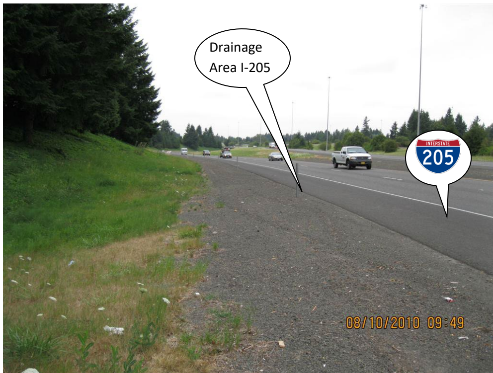
Photo 1: Drainage area to the facility looking to the west or decreasing mileage.
