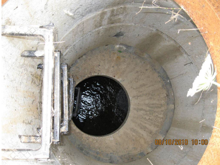
Photo 4: The inlet vault structure on the northwest end of the facility.
