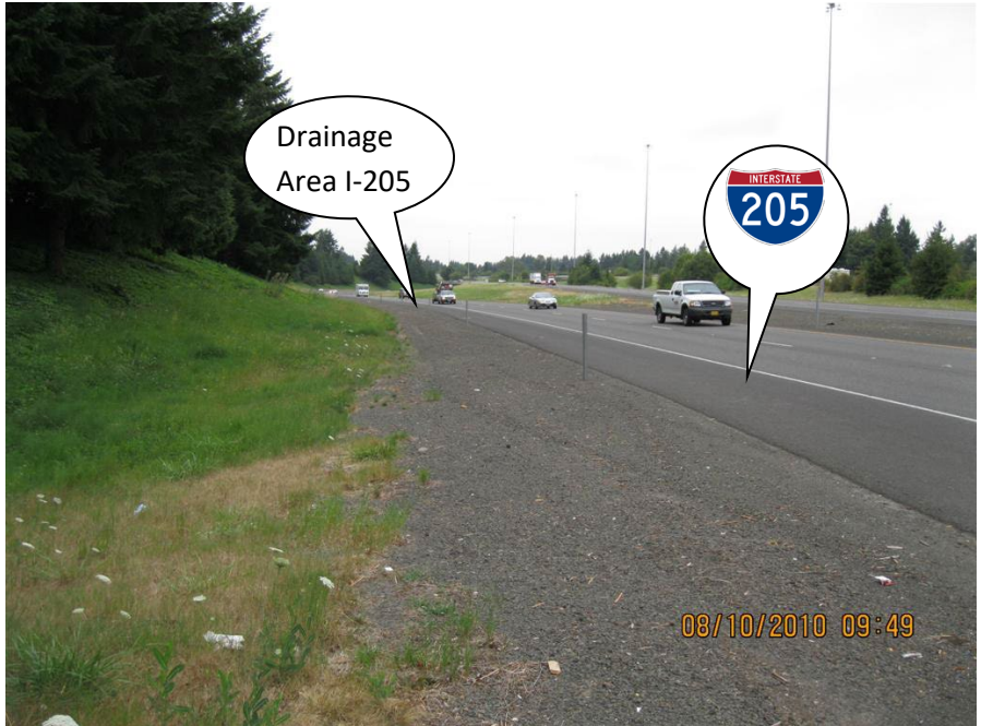
Photo 1: Facility Drainage area looking west or decreasing mileage.
