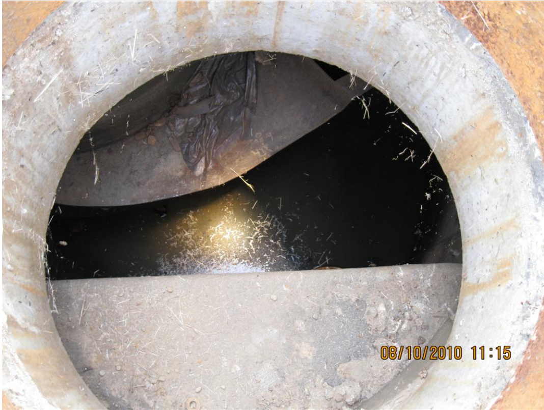
Photo 3: Water quality manhole interior
