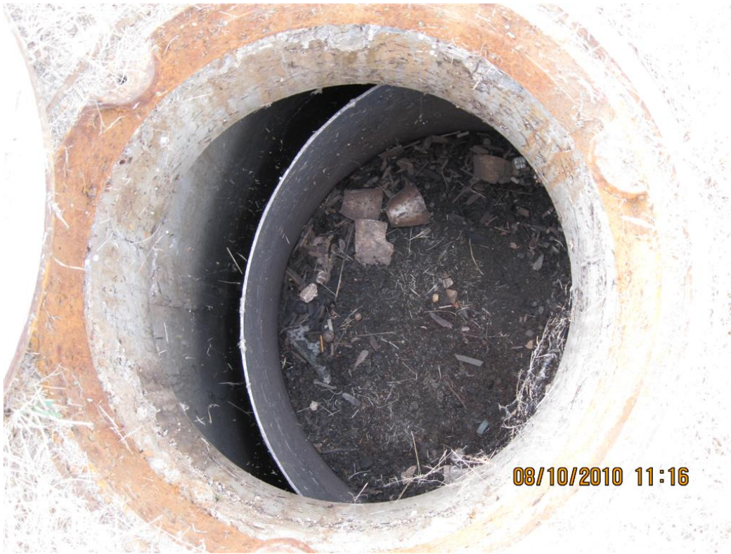
Photo 2: Water quality manhole interior
