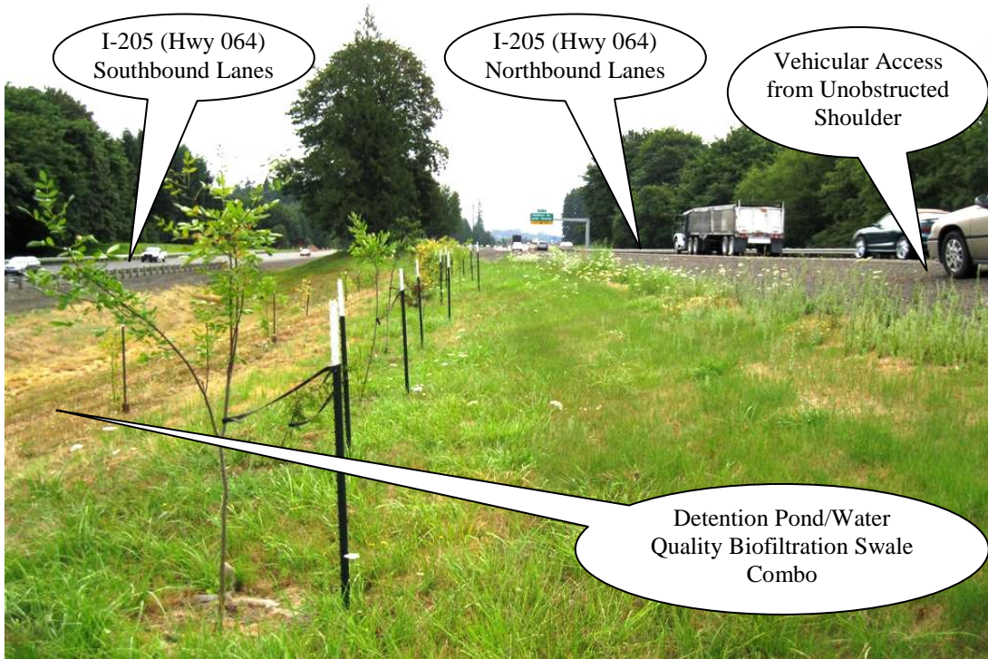
Photo 1: Overview of the facility. Photo taken facing east. Vehicular access from unobstructed shoulder of northbound lanes of I-205 (Hwy 064.)
