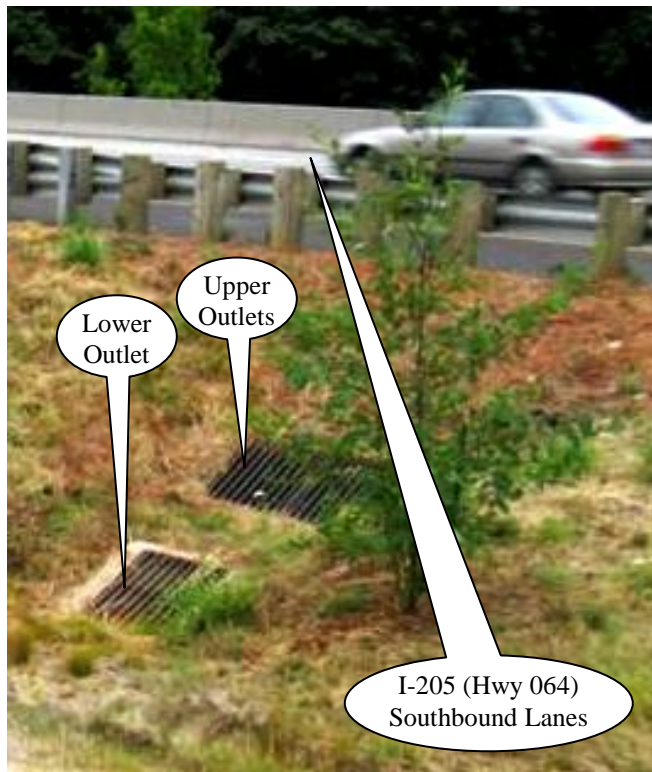
Photo 3: Facility outlet structures
