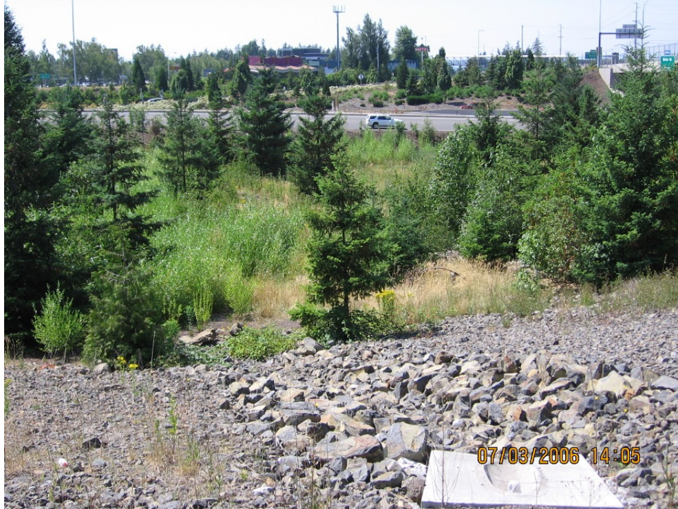
Photo 3: Outlet for water quality swale (Point E, Operational Plan), discharging into the adjacent detention facility to the west (DFI D00085).
