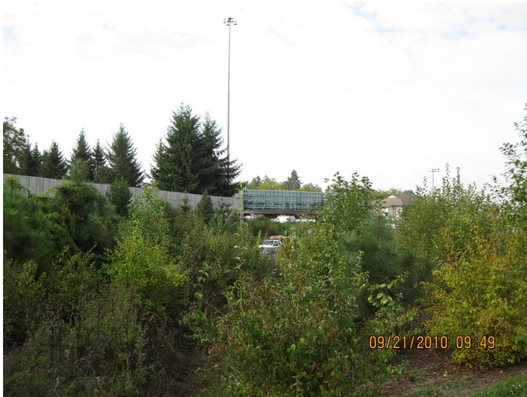
Photo 2: Water quality biofiltration swale.
