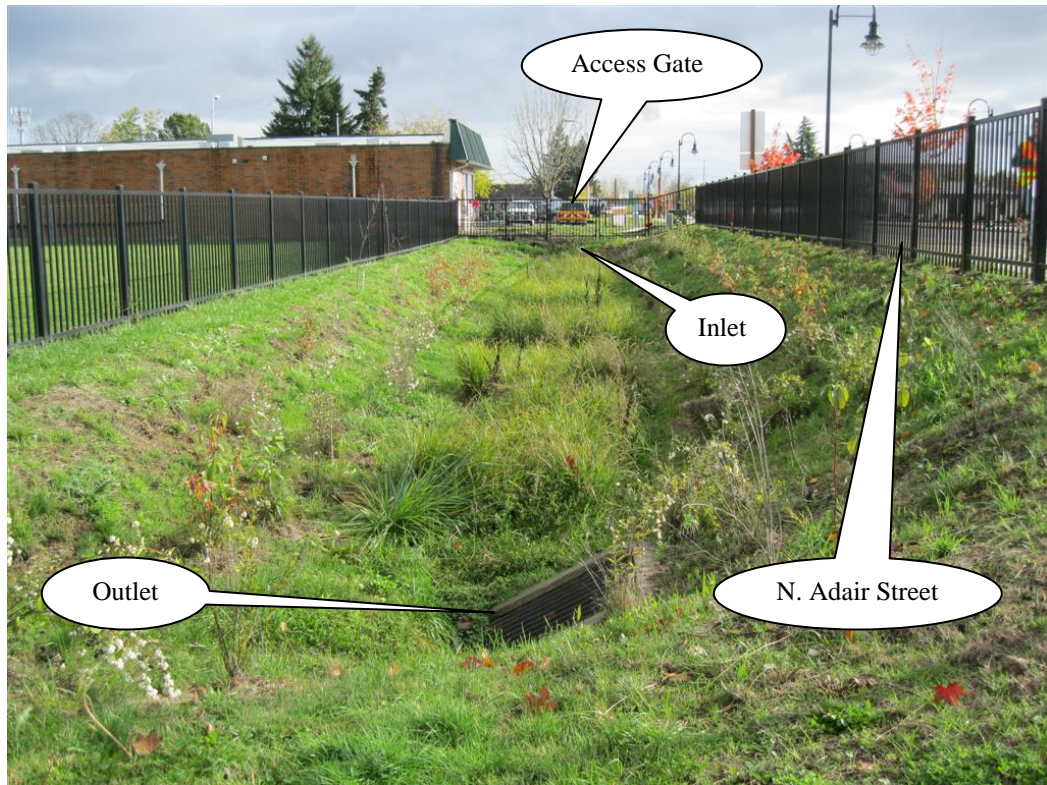
Photo 1: This is an overview of the swale looking towards the East.
