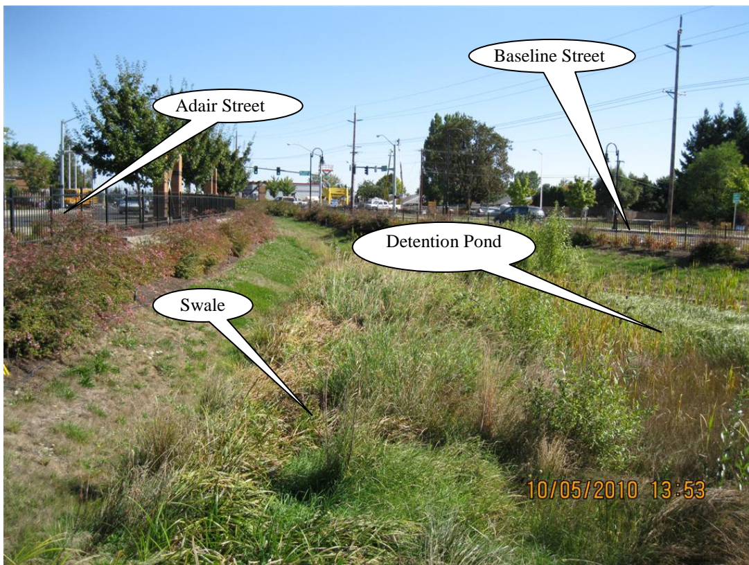
Photo 1: Detention Pond/ WQ Swale Combo Looking East
