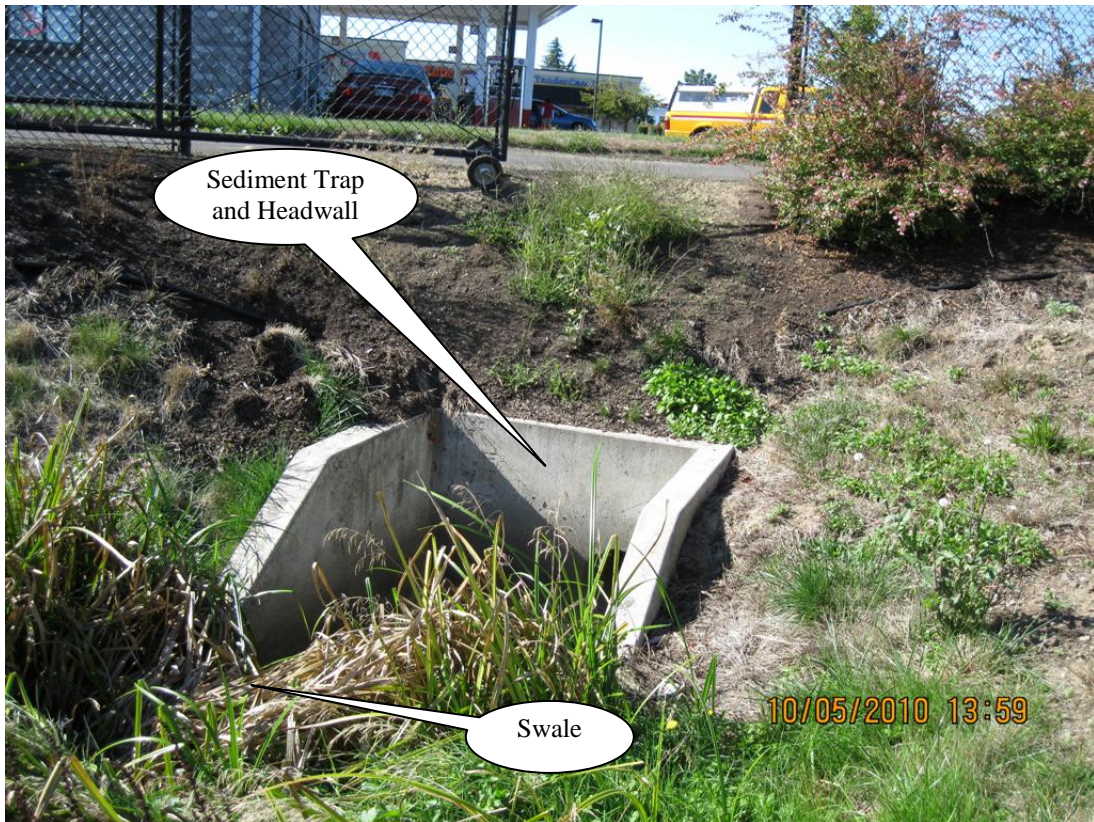
Photo 3: Swale Inlet Looking West
