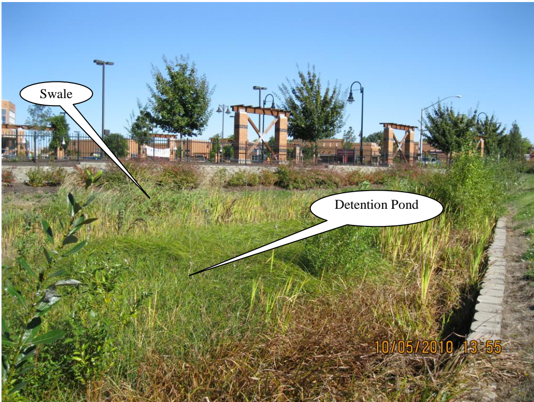
Photo 4: Detention Pond Looking East
